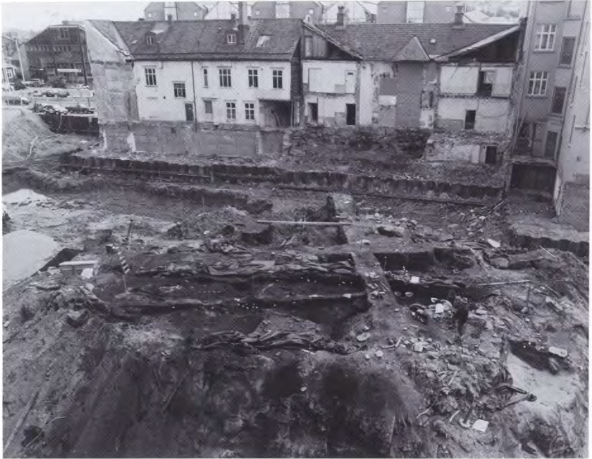
F-site under excavation; looking East.
