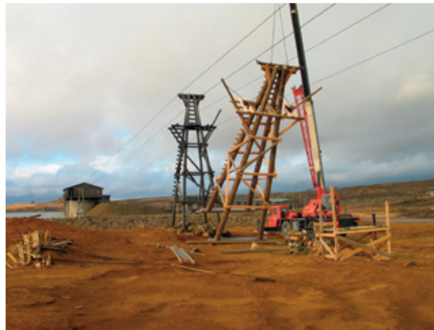
63: Restoration of the cableway – raising a new pylon.
