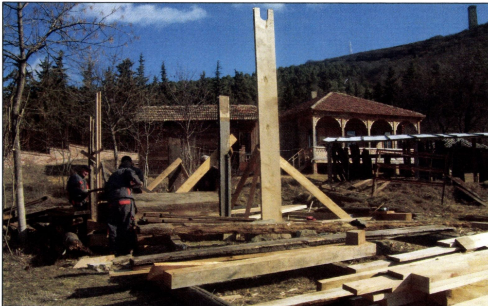
Restoration has been started
