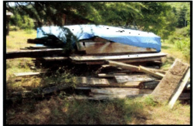
Usable and restorable authentic timber of the Nigvziani house
