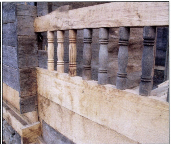
Mixing authentic and new timber on Nigvziani house
