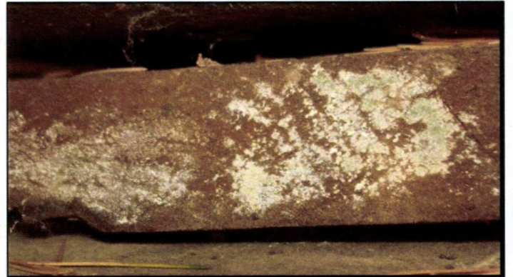
Example of the bio-deteriorated boards
