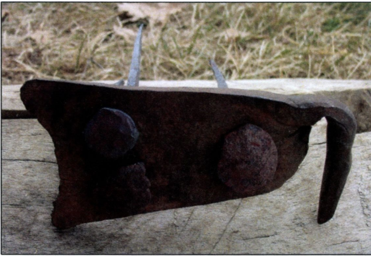
An old door steel detail
