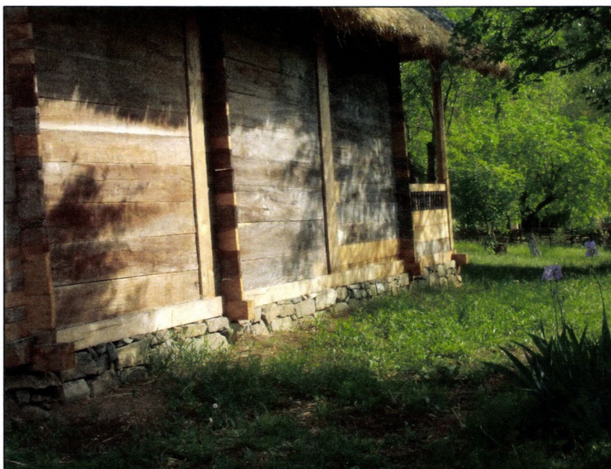
"Nigvziani" cooking House after restoration
