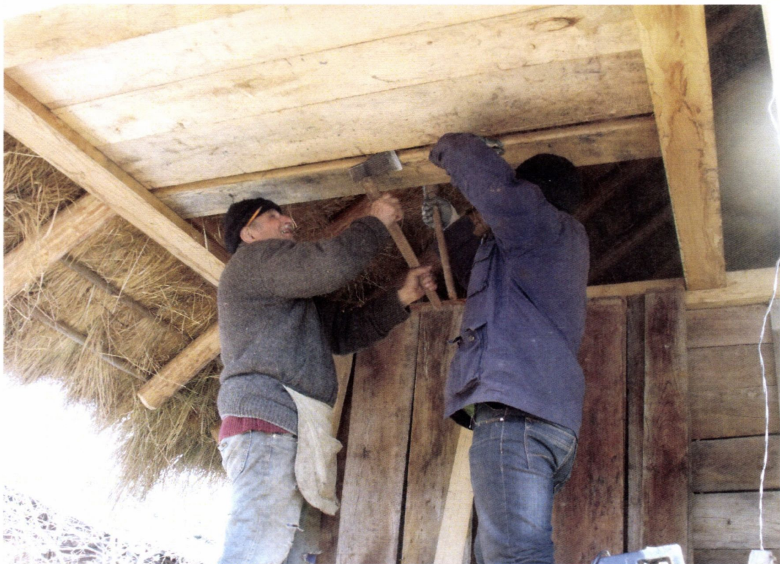
Boarding the ceiling of the balcony of "Nigvziani"
