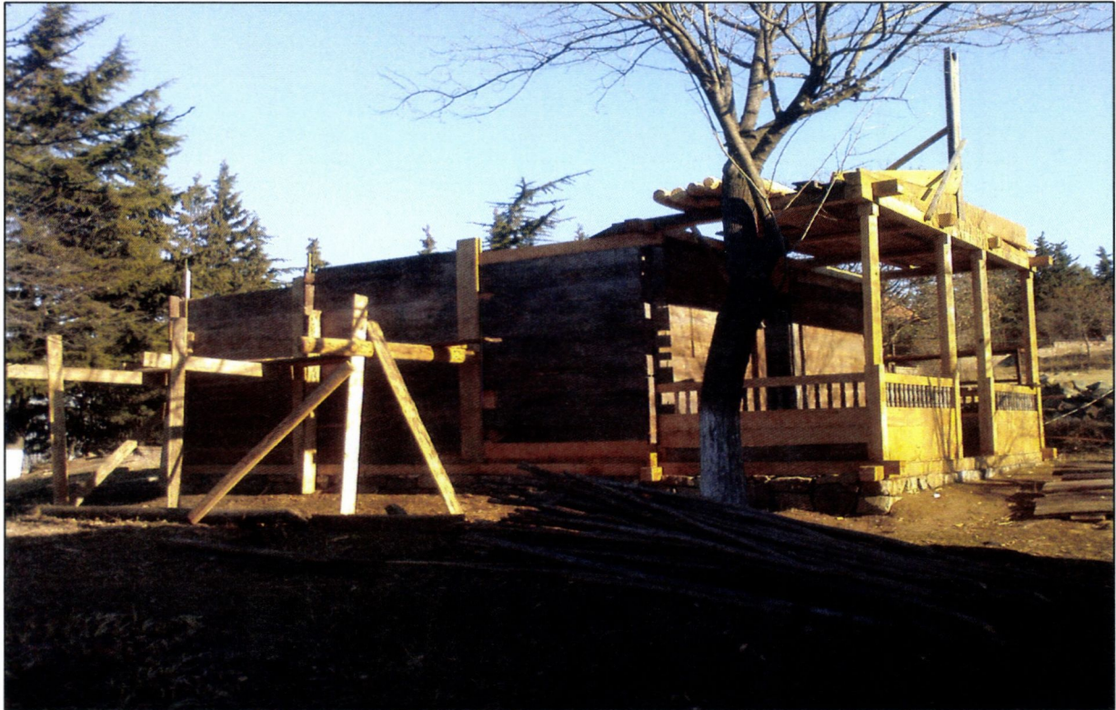
Nigvziani House before starting the roofing works
