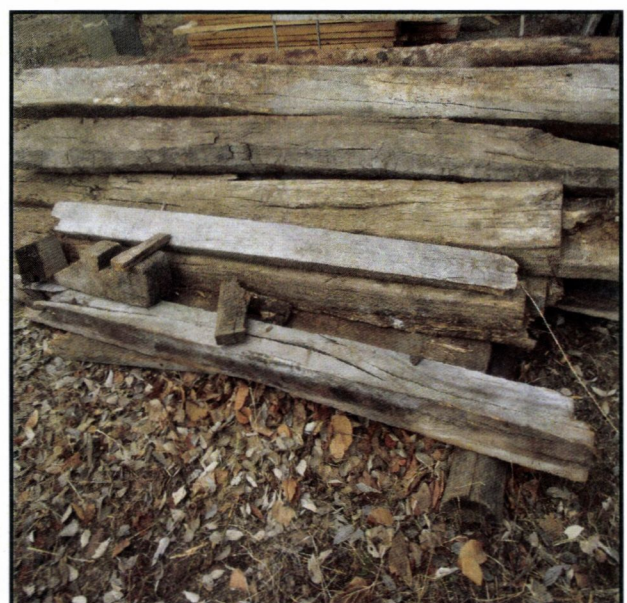
Sample of unusable authentic timber of the Nigvziani house
