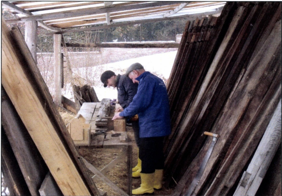
Selecting usable timber from authentic materials before starting restoration
