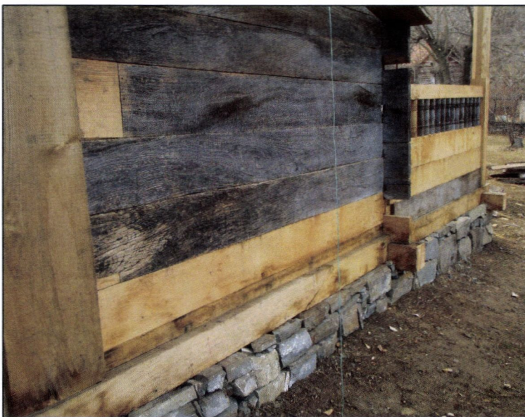
Mixing authentic and new timber on Nigvziani house
