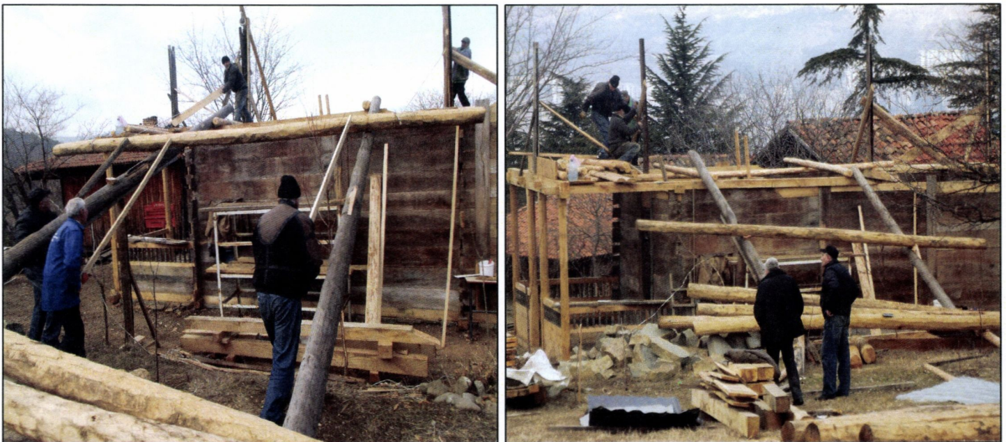
Using traditional way of lifting and mounting wooden logs
