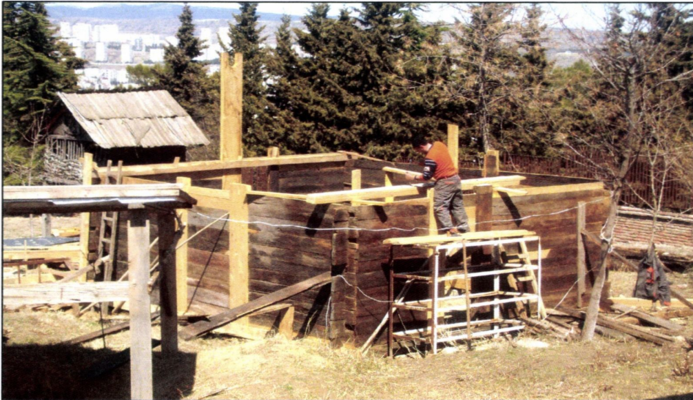
Finalizing the walls
