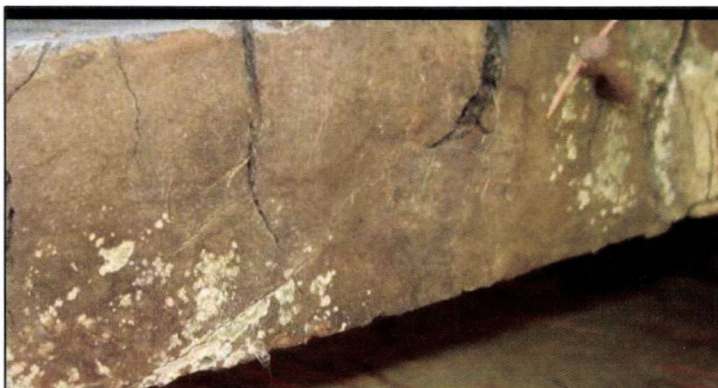
Example of the bio-deteriorated boards
