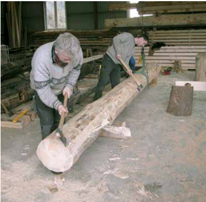
Making a new post. From the left, Erlend Gjelsvik and Stig Nordrumshaugen. Photo: Ellen Devold 2005.
