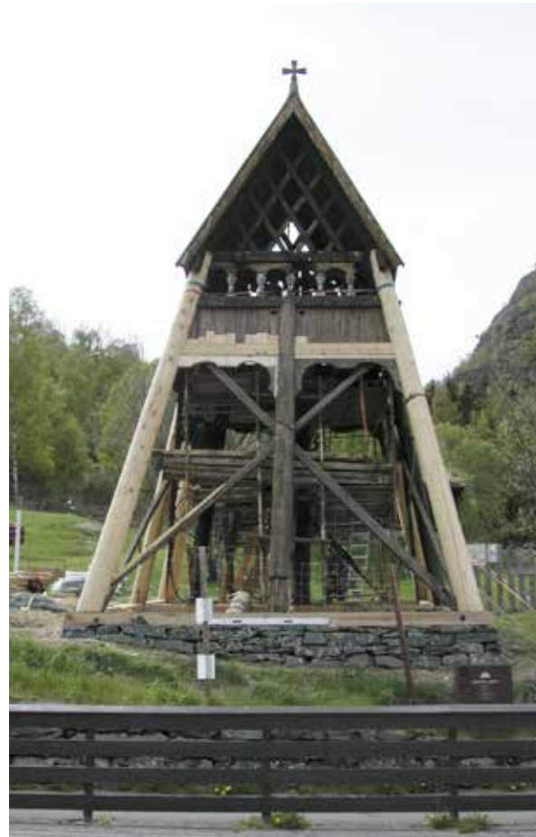
The bell tower viewed from the east, after the repairs to the load-bearing structure had been completed, and before it was panelled. Photo: Ellen Devold 2006.
