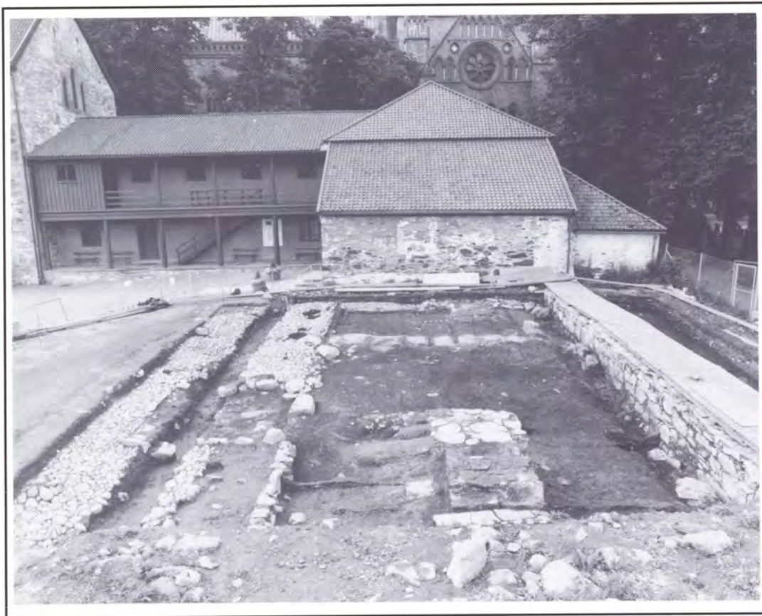
Fig. 27 BUILDING I, Herrehuset (looking N.)
