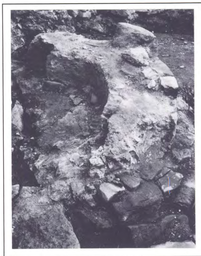
Fig. 45. NIDARHOLM ABBEY CHURCH. Plate showing the interior and foundation of the apse. Looking N.
