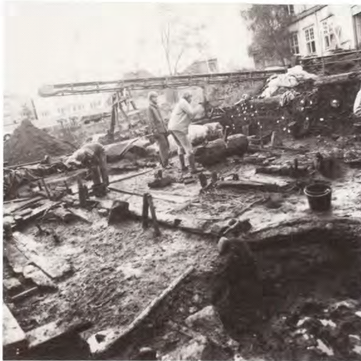
Fig. 3. From the excavation of areas FH and FF 1976. (Photo RA 1985).
