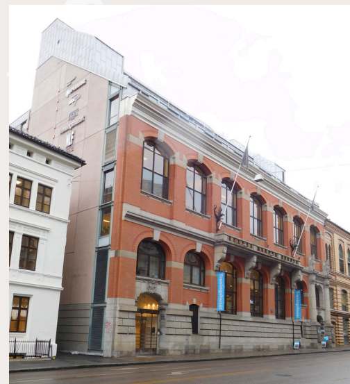
Turnhallen in Oslo exemplifies heritage protection values linked to experiential values. Following a fire in 1988 that gutted the interior of the building, a new building was erected behind the preserved facade. Photo: Directorate for Cultural Heritage
