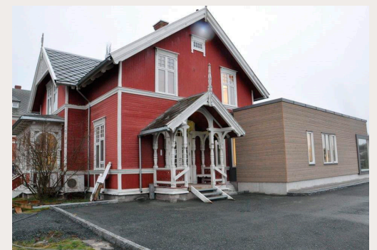
An extension in Levanger which severely impairs the heritage value of the former school principal’s residence. Photo: Trond Blikø/Trønderavisa
