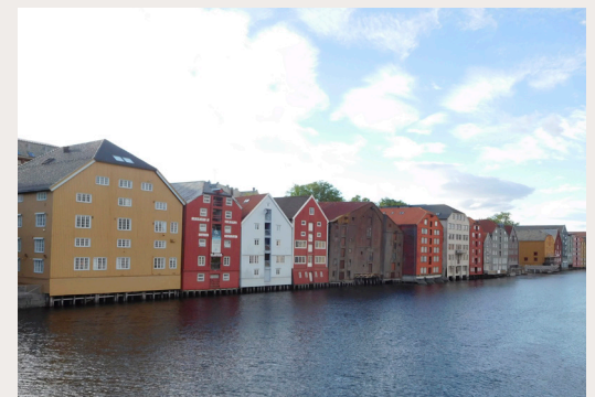
The piers in Trondheim. This row of buildings has immense national value, but their future use poses a challenge. Photo: Directorate for Cultural Heritage
