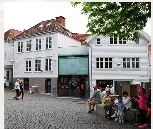
Godt Brød AS at Sølberget, Stavanger. Arkitekt Helen & Hard. A good example of an infill project in which the compact newbuild offers a positive contrast to the adjacent buildings while being lesser in volume. Photo: Siv Egeli, Stavanger Local Authority
