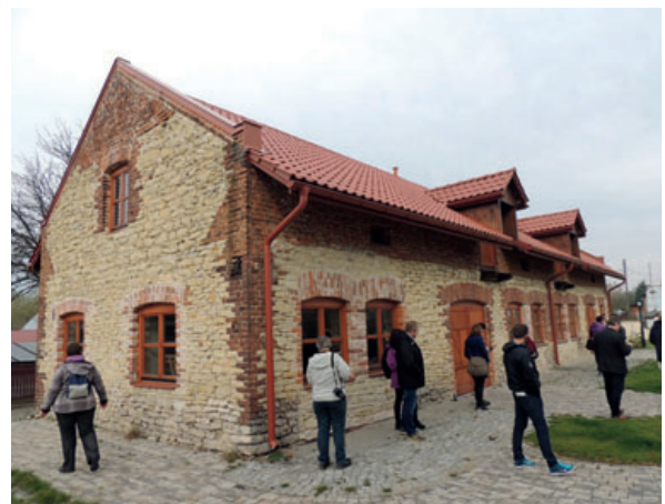
The former parish utility building in Narol; after renovation it was used as a social therapy centre, photo by M. Hejnowicz, private archive
