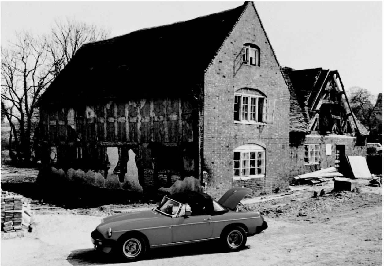
Figure 2.1 Brookgate Hall, Plealey, is one of the oldest manor houses on the Shropshire border between England and Wales. The earliest part was built in 1350. In 1500 a wing was added. In 1612, part of the medieval structure was destroyed and a new parlour built. Photo before the restoration 1987-1990 by the architect and owner, Graham Moss. The house had been empty for several years, the roofs were leaking and the house was in a bad state of repair. (Photo by Graham Moss).
