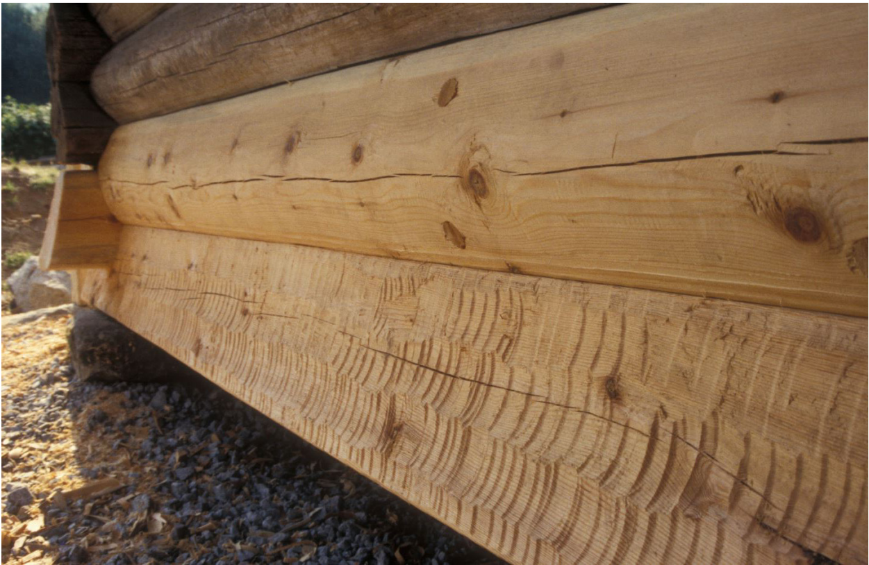
Figure 5.8 A sill beam prepared using spret-telgjing .
