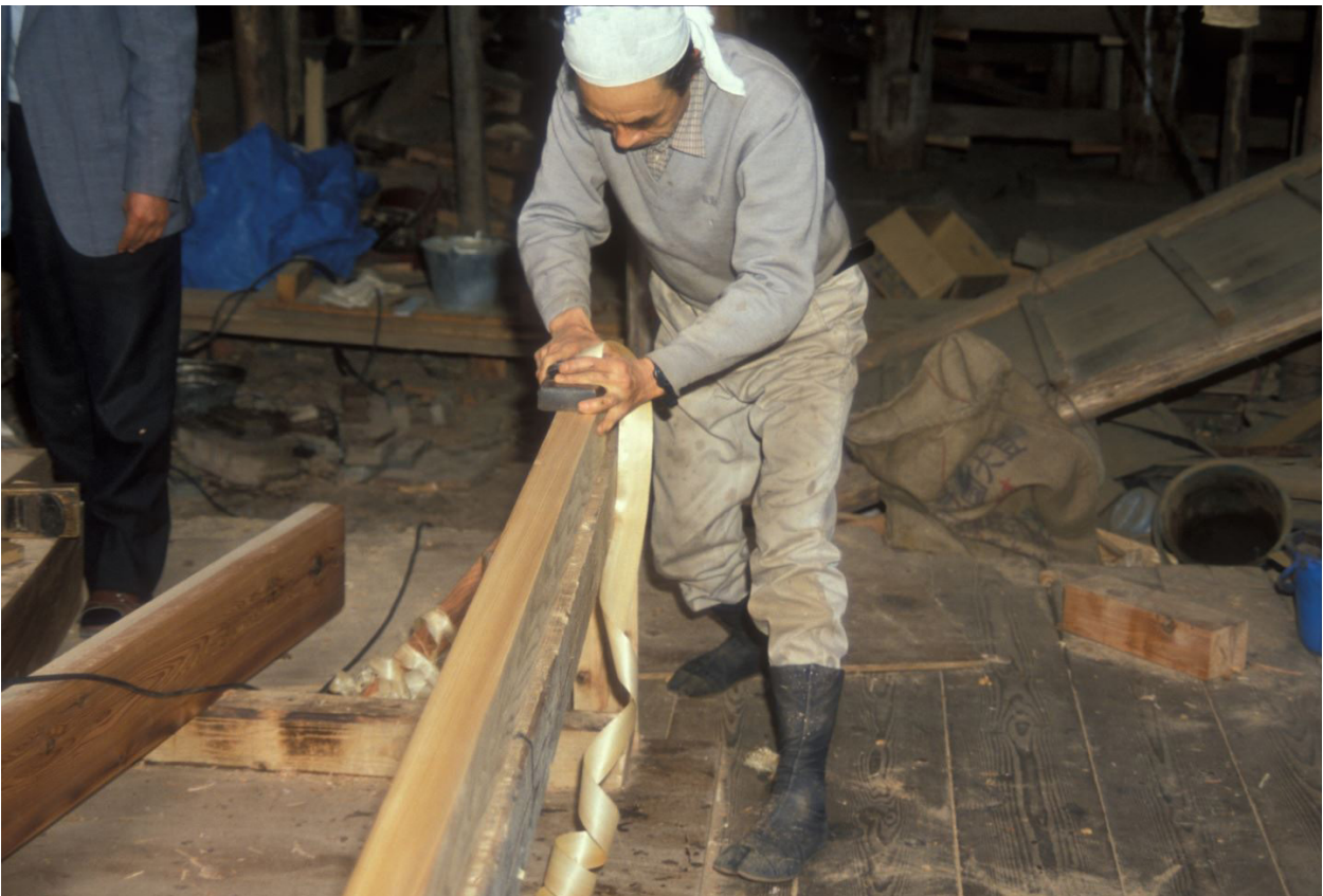
Figure 5.7 Carpenter at the repair site of the three-storied pagoda of Oyama-dera, Ibaraki, Japan in 1989. planing. The long, perfect shaving is a trademark of the excellence of Japanese carpentry work. The carpenter is pulling the plane.
