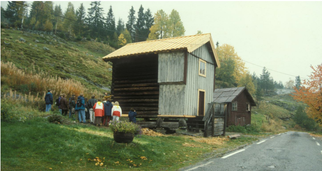
Figure 5.9 A repaired medieval timber building in Tokke, Norway. Only minor repairs have been made to the log-structure. The roof boarding has been completely renewed.
