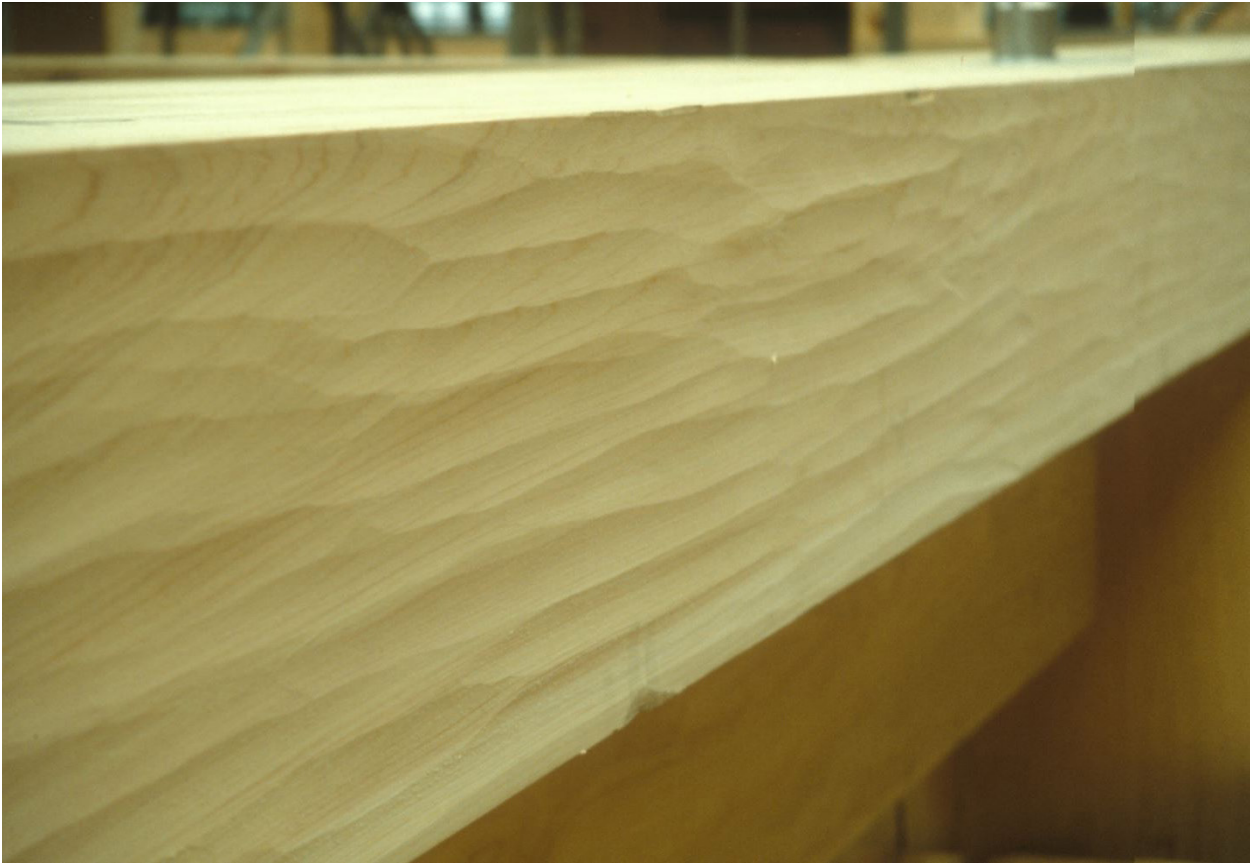
Figure 5.4 Surface of a beam of Japanese cypress ( Chamaecyparis obtusa ) prepared using the yari-ganna .
