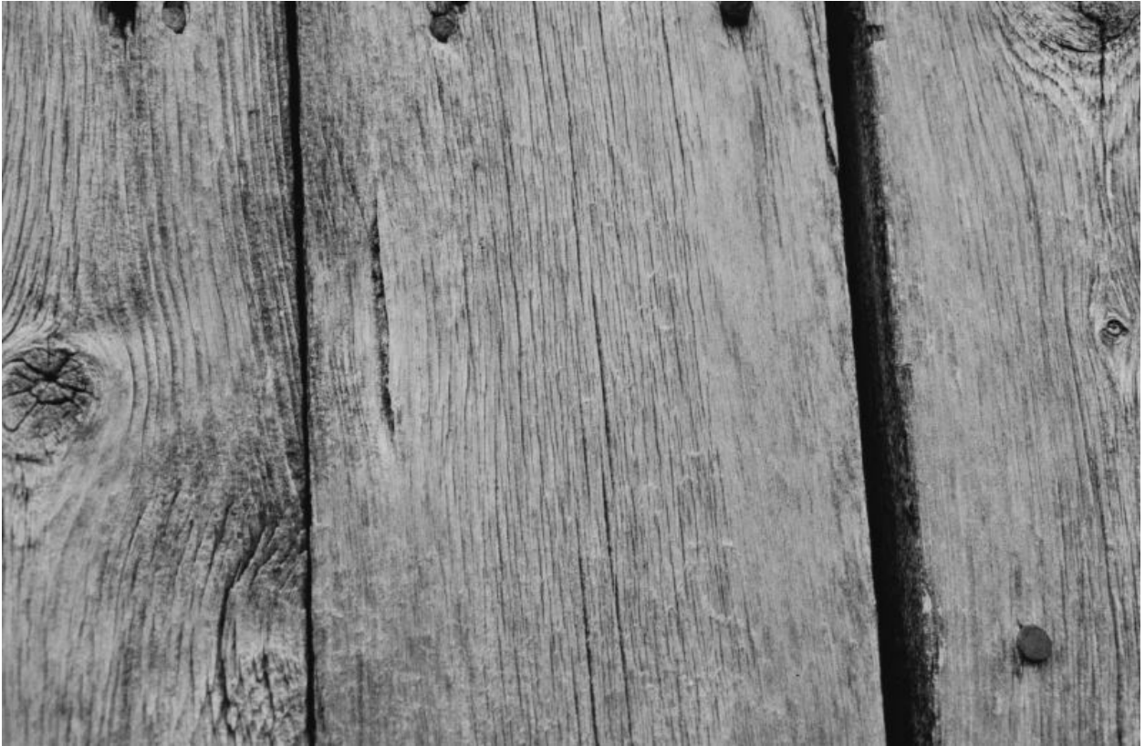
Figure 8.5 External boarding of aspen ( Populus tremula ), about 80 years old. This external boarding has never been treated with paint or coating. It is still in excellent condition, despite being on an exposed site.
