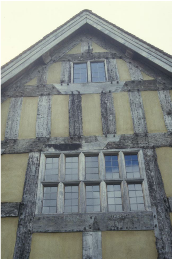
Figure 2.3 Brookgate Hall after restoration. Detail of a gable showing replaced timber in the frame. Brookgate Hall after restoration. Detail of a gable showing replaced timber in the frame.
