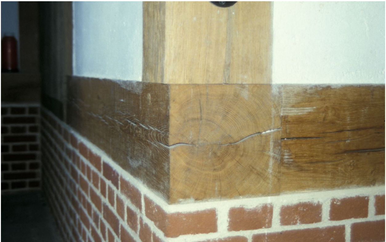
Figure 8.3 Shakespeare's Globe, London (1997). Oak heartwood ( Quercus robur ) was used in all external (exposed) members, although the architect and builder Peter McCurdy reckoned that the original structure probably contained timber with a high proportion of sapwood.
