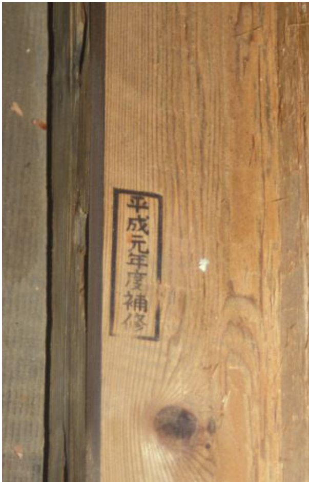
Figure 4.8 New members or parts of members should have the date of the repair inscribed on them so that they can be identified later. Here is an example from Japan where the date of the repair is burnt into the wood. The characters mean Heisei gannen go hoshu, that is: this piece of timber was put into the structure in 1989, the first year of the Heisei era.
