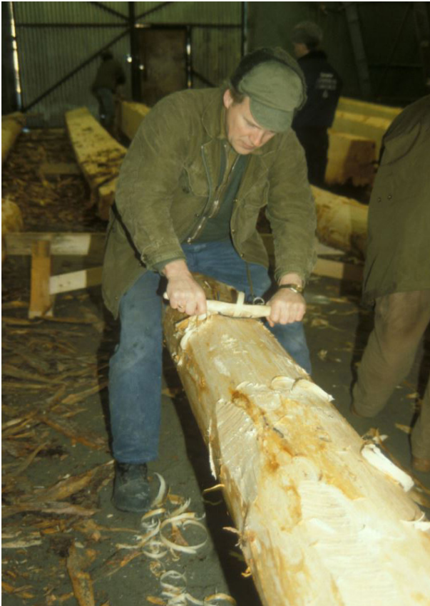
Figure 5.6 Carpenter planing a log with a spokeshave.
