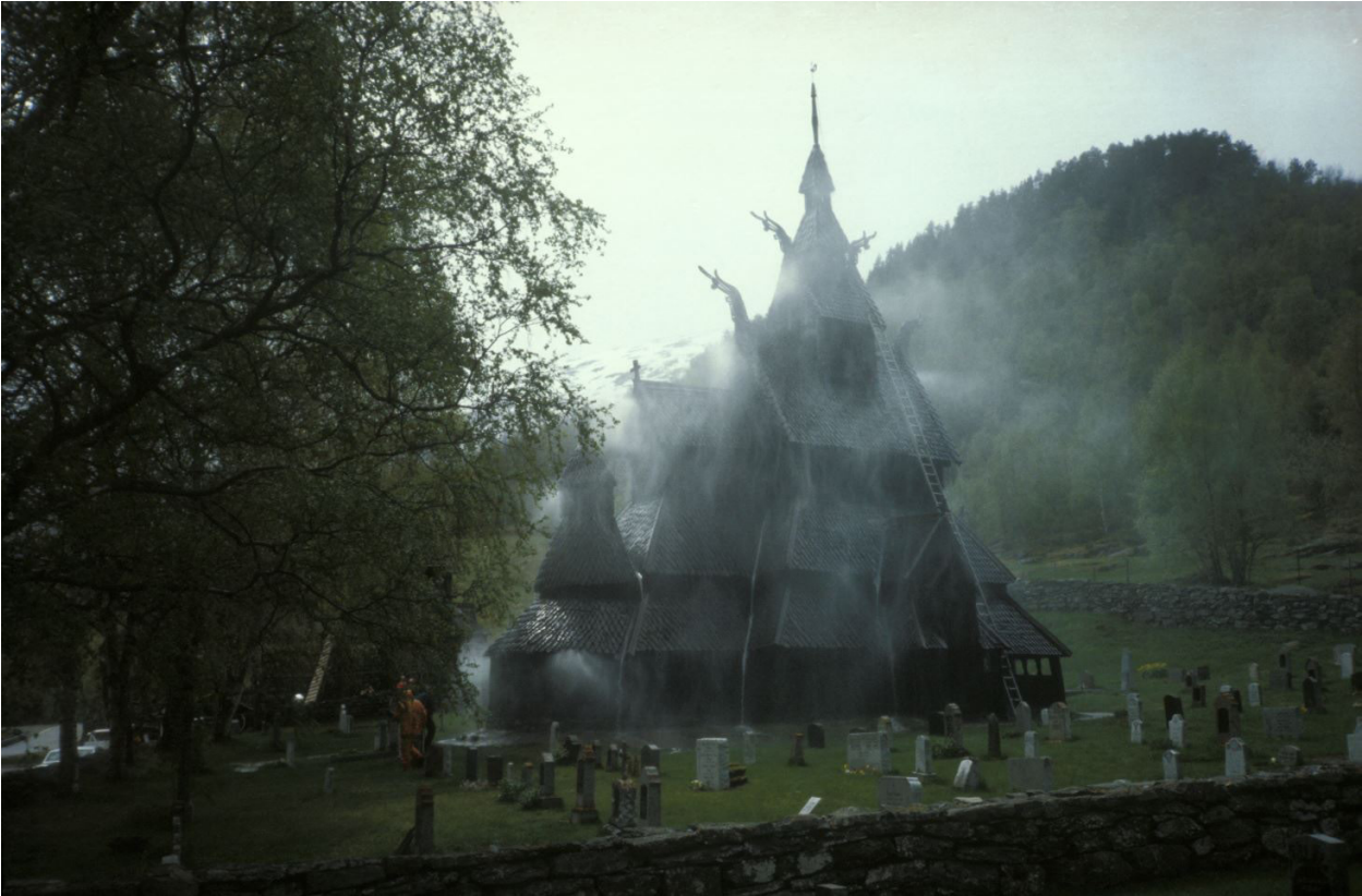
Figure 7.16 Borgund stave church, Sogn, Norway, during a sprinkler fire extinguishing system test in 1982. All the 28 medieval stave churches have fire detection and fire extinguishing systems. Traditional sprinkler systems and advanced mist systems are used.
