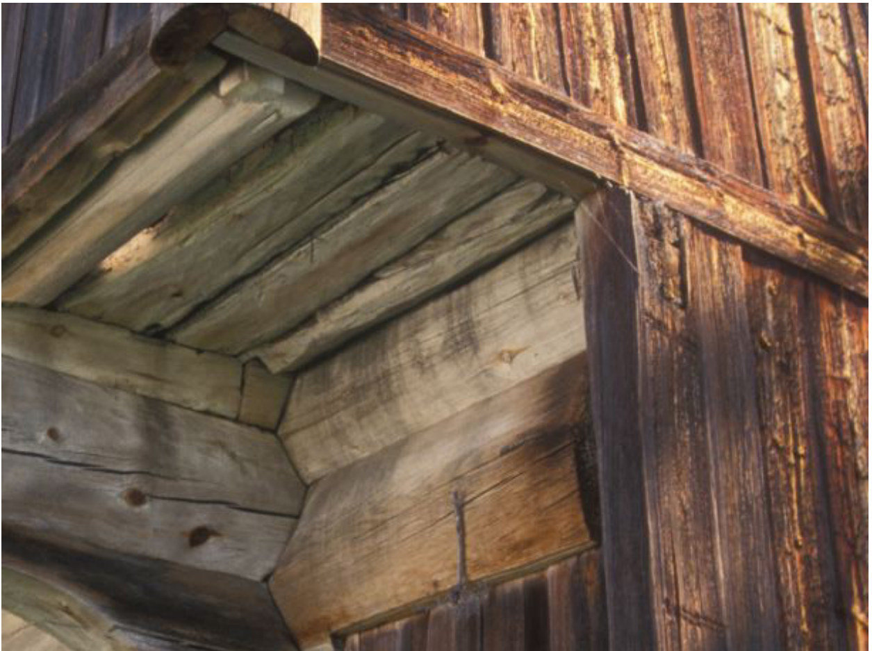
Figure 8.10 A medieval timber structure in Telemark, Norway. The medieval logs which have not been exposed to the weather are grey in colour and look like new timber. The external boarding which is secondary, is dark brown in colour and has eroded due to weathering.
