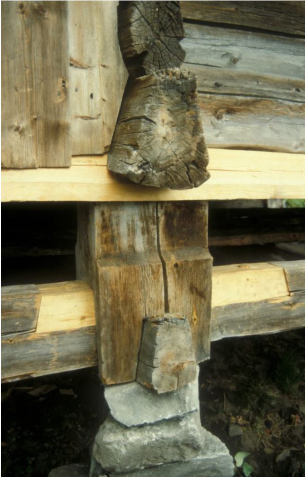
Figure 5.10 Repairing a medieval storehouse in Tokke, Norway. The structure is repaired in situ without dismantling. New, well-seasoned wood is jointed in.
