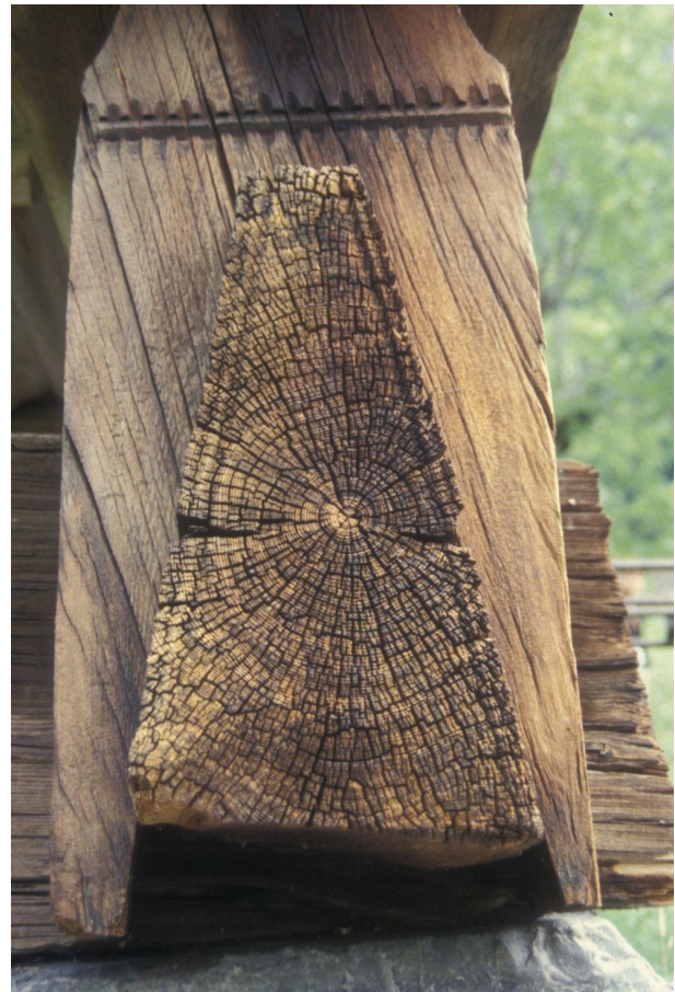
Figure 8.8 Detail of the sill-beam in a Norwegian log-structure from late eighteenth century. Note the extremely narrow width of the annual rings, and that the sapwood content is insignificant. It is very well preserved, despite exposure to the elements over two centuries.
