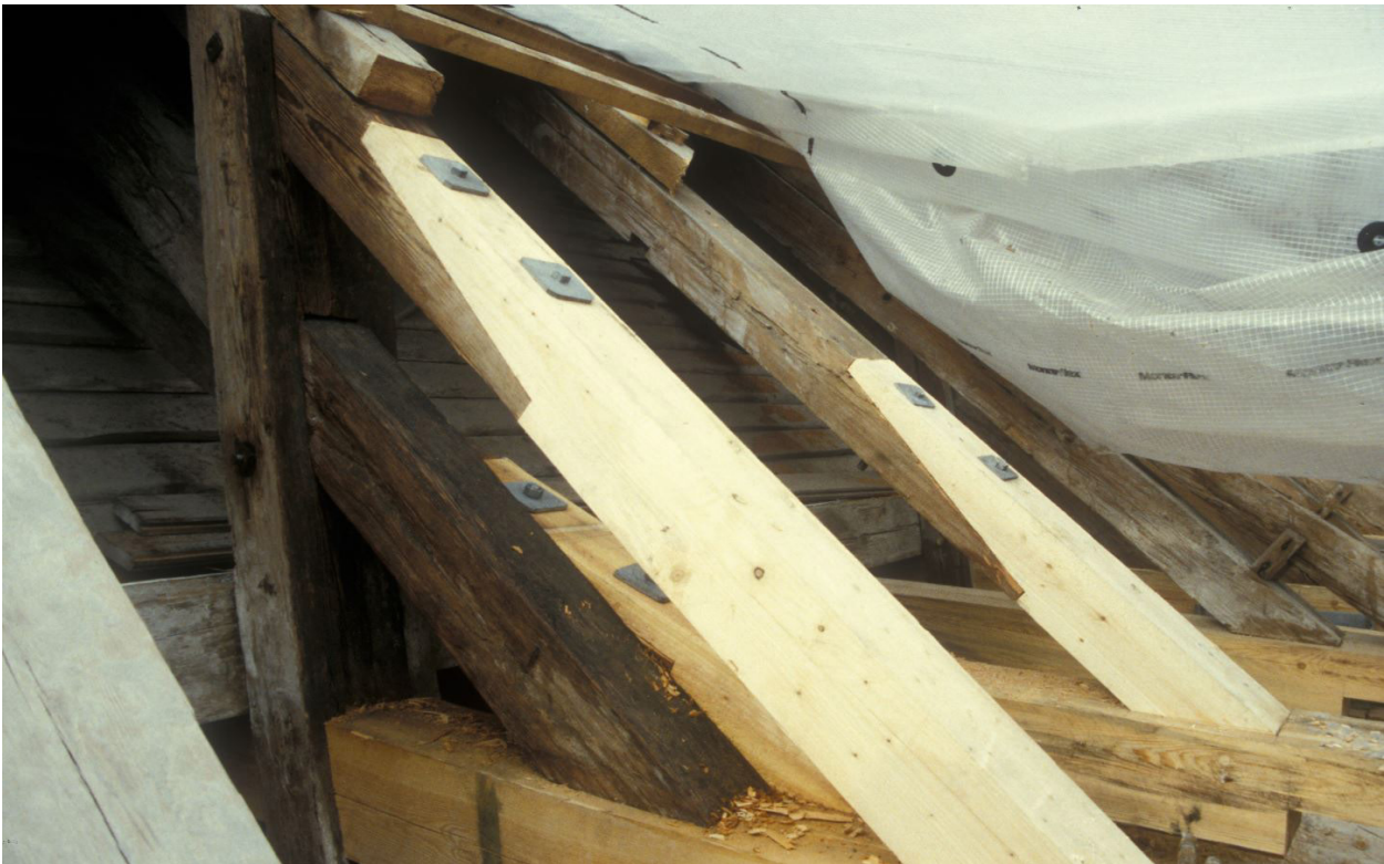
Figure 4.1 Hørsholm church outside Copenhagen, Denmark. Repair of rafters 1997. New and old timber is jointed and the joint reinforced with steel bolts and toothed-plate connectors.
