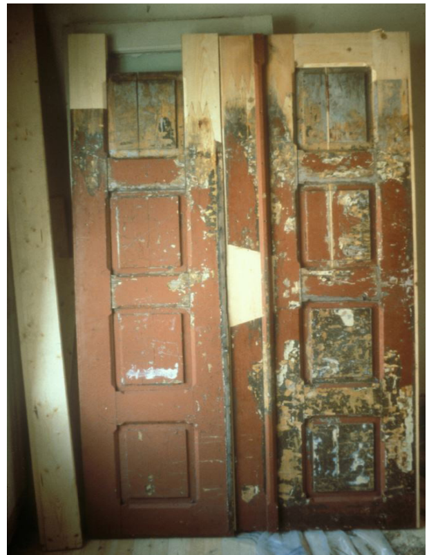
Figure 4.12 Pieced-in repair of a door. Mosjøen, Norway.
