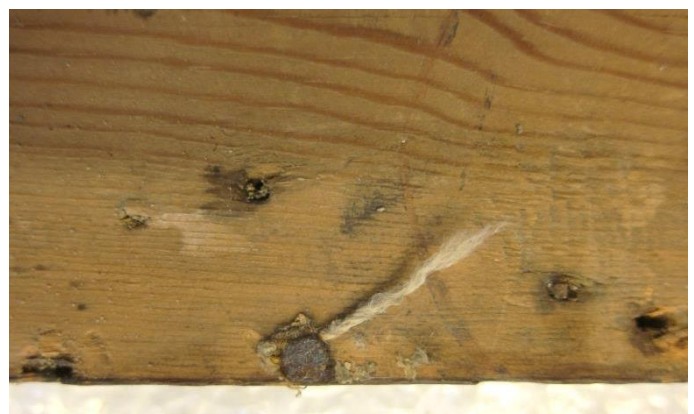
Figur 7. Eldre monteringshuller langs ytterkanten
