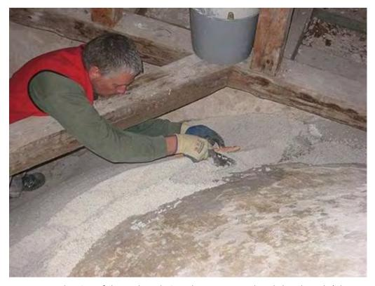
Figure 3. Application of thermal insulation plaster on a medieval church vault (photo: Poul Klenz Larsen)
