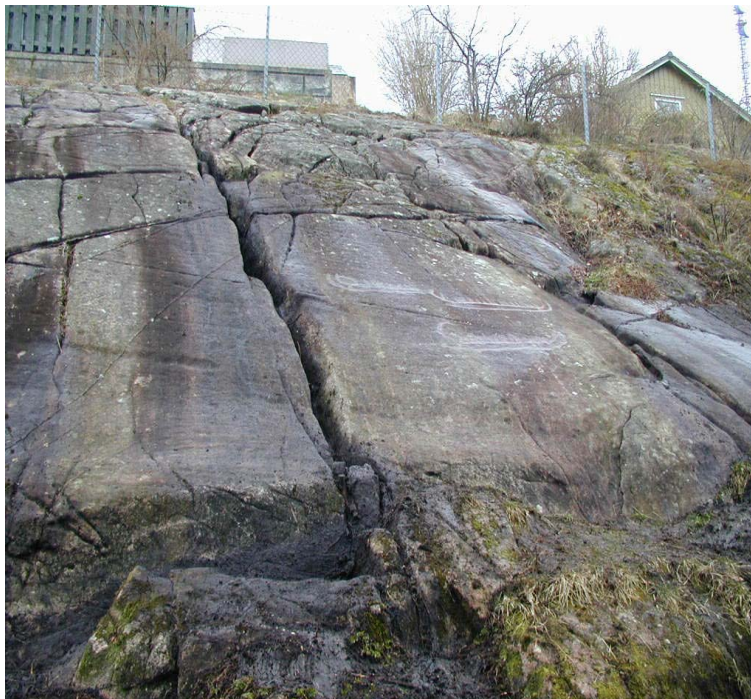
Figure 51. B) After cleaning of vegetation in cracks at Husabø, Egersund, Rogaland. Photo: AmS.
