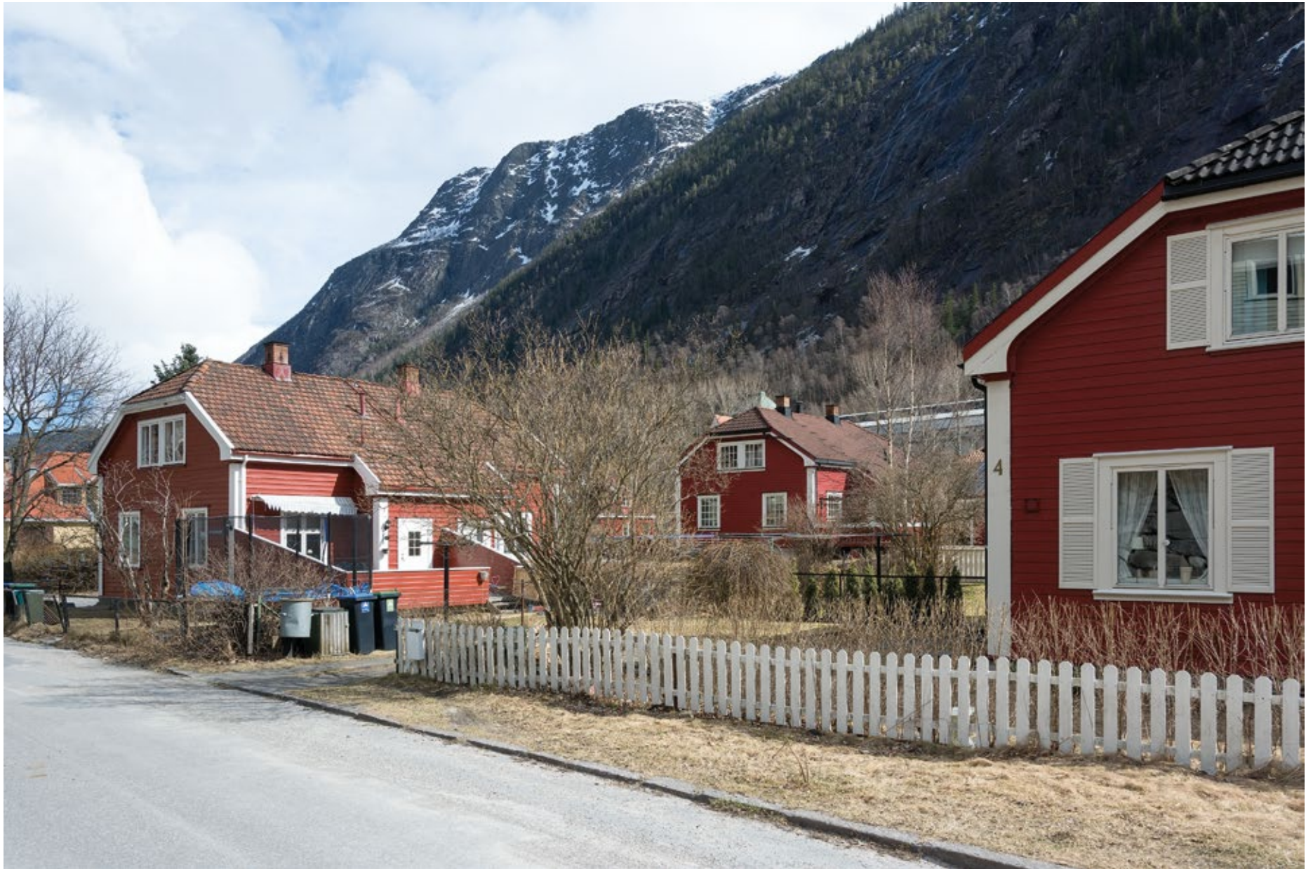
Fig. 101 Rødbyen housing area, Rjukan Hydro Town Photo: Per Berntsen
