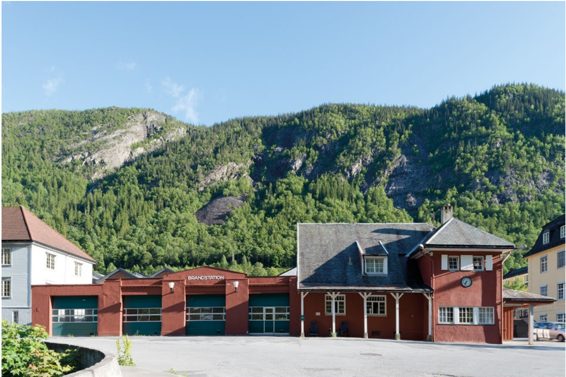
Fig. 99 Gatehouse and fire station, Rjukan Hydro Town. Photo: Per Berntsen
