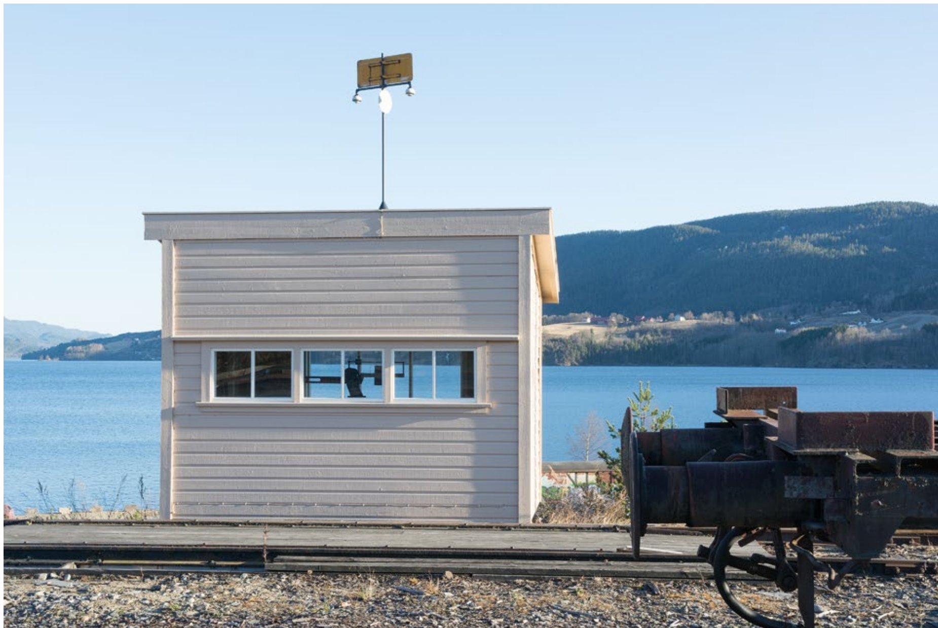
Fig. 64 Wagon weighing hut at Notodden Railway Station. Photo: Per Berntsen
