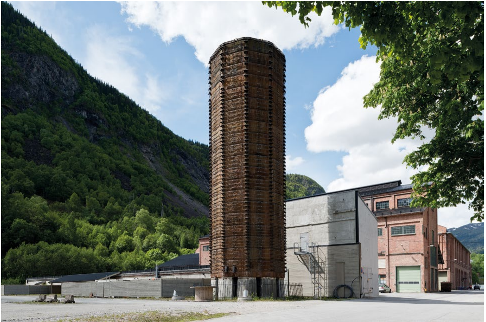
Fig. 60 Acid Tower, Hydro Industrial Park in Rjukan. Photo: Per Berntsen
