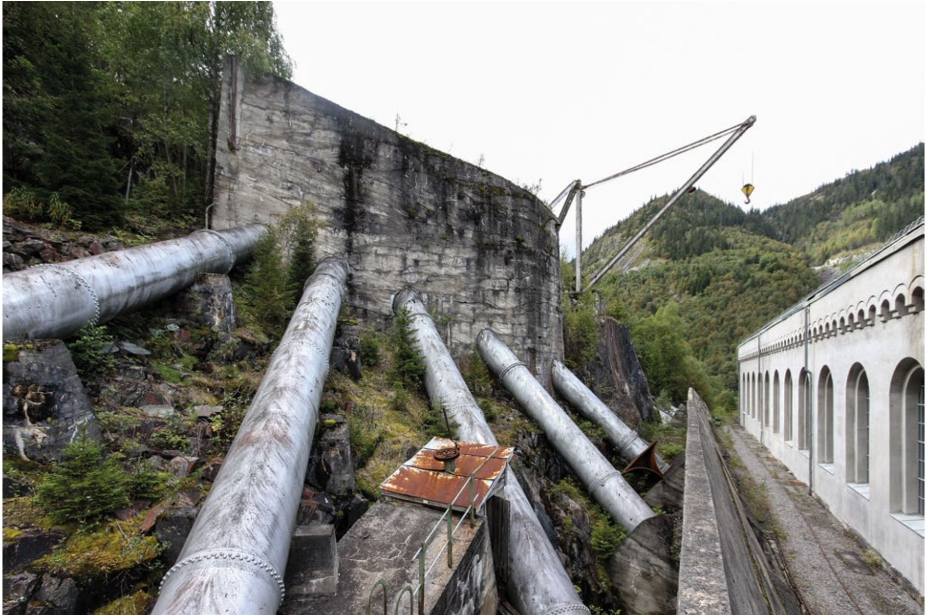
Fig. 22 Penstock and Vemork railway track at Vemork Power Plant. Photo: Eystein M. Andersen
