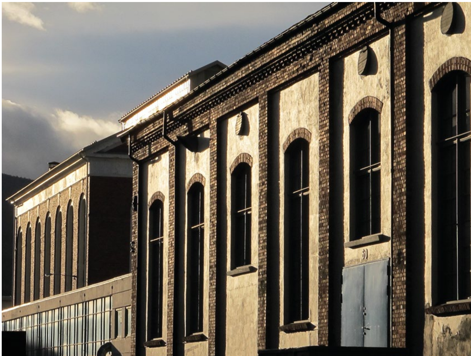
Fig. 44 Furnace House A, Hydro Industrial Park in Notodden. Photo: Trond Taugbøl
