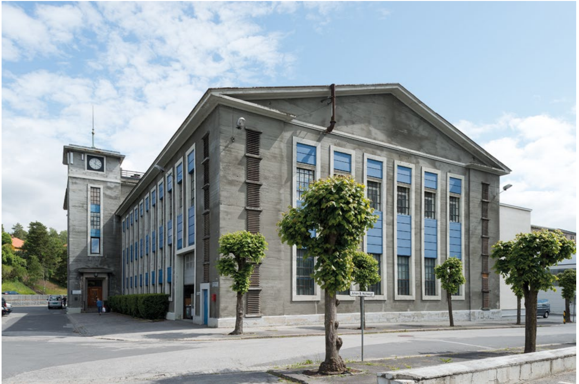
Fig. 48 Hydrogen Plant, Hydro Industrial Park in Notodden. Photo: Per Berntsen
