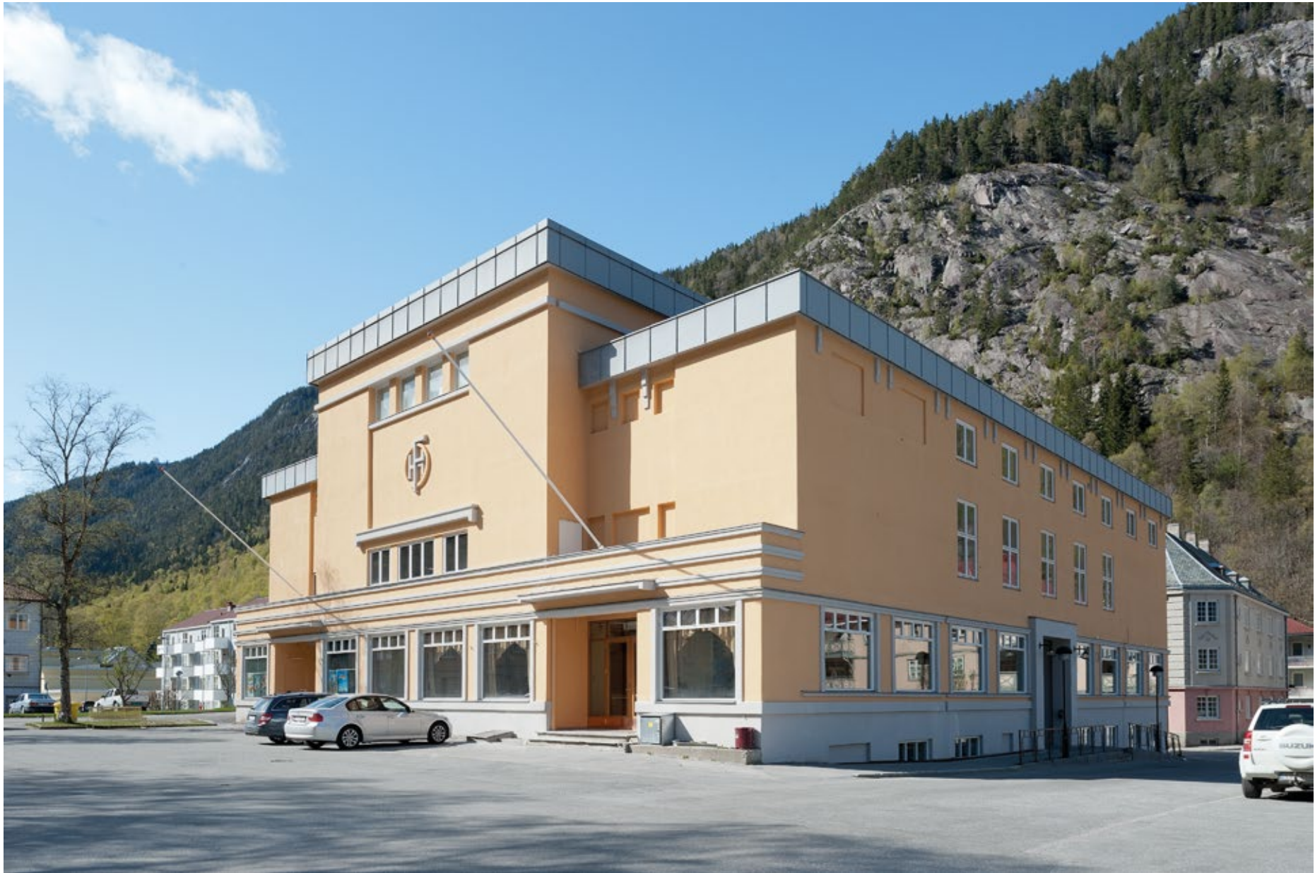
Fig. 103 The Rjukan House, Rjukan Hydro Town. Photo: Per Berntsen
