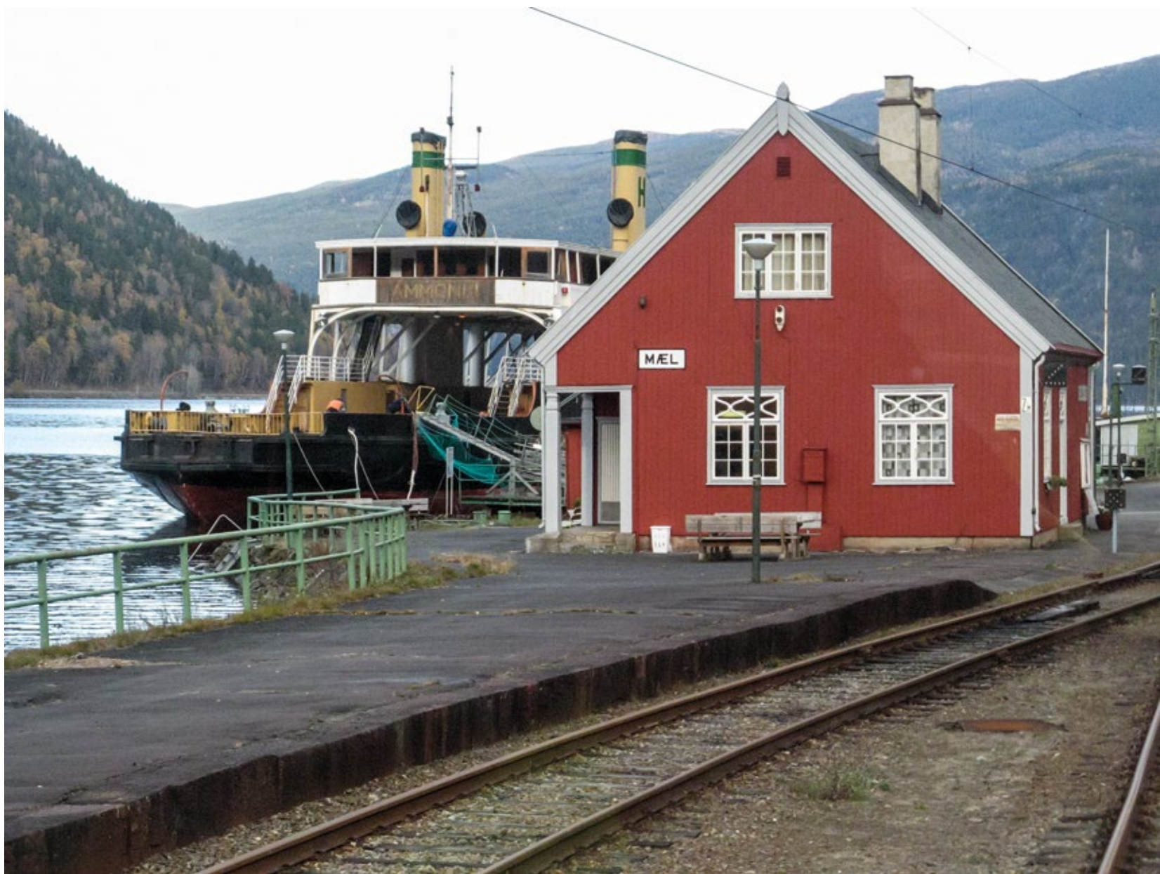
Fig. 79 Mæl Railway Station Building and D/F Ammonia. Photo: Trond Taugbøl
