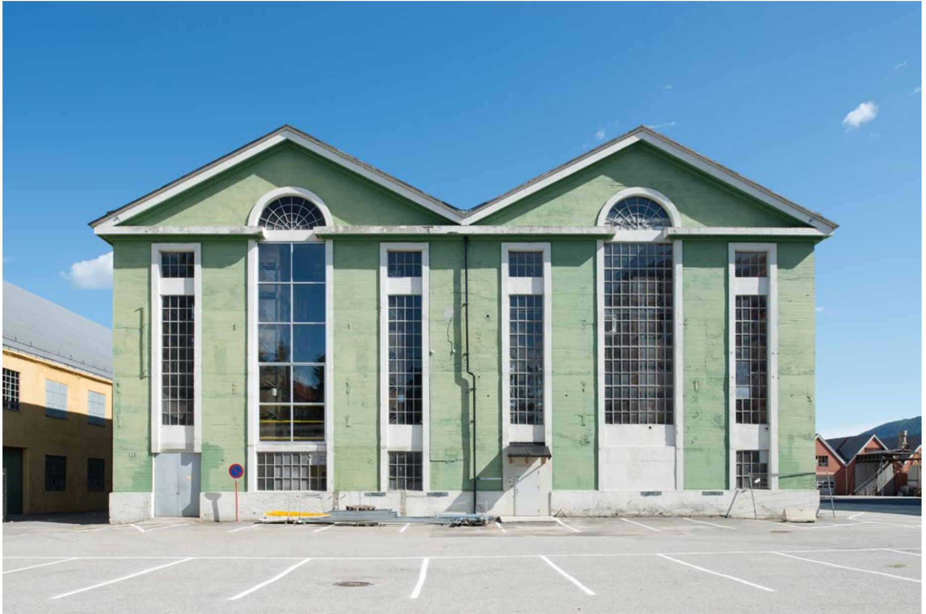
Fig. 50 Nitrogen Plant and Gas Cleaning Plant, Hydro Industrial Park in Notodden. Photo: Per Berntsen
