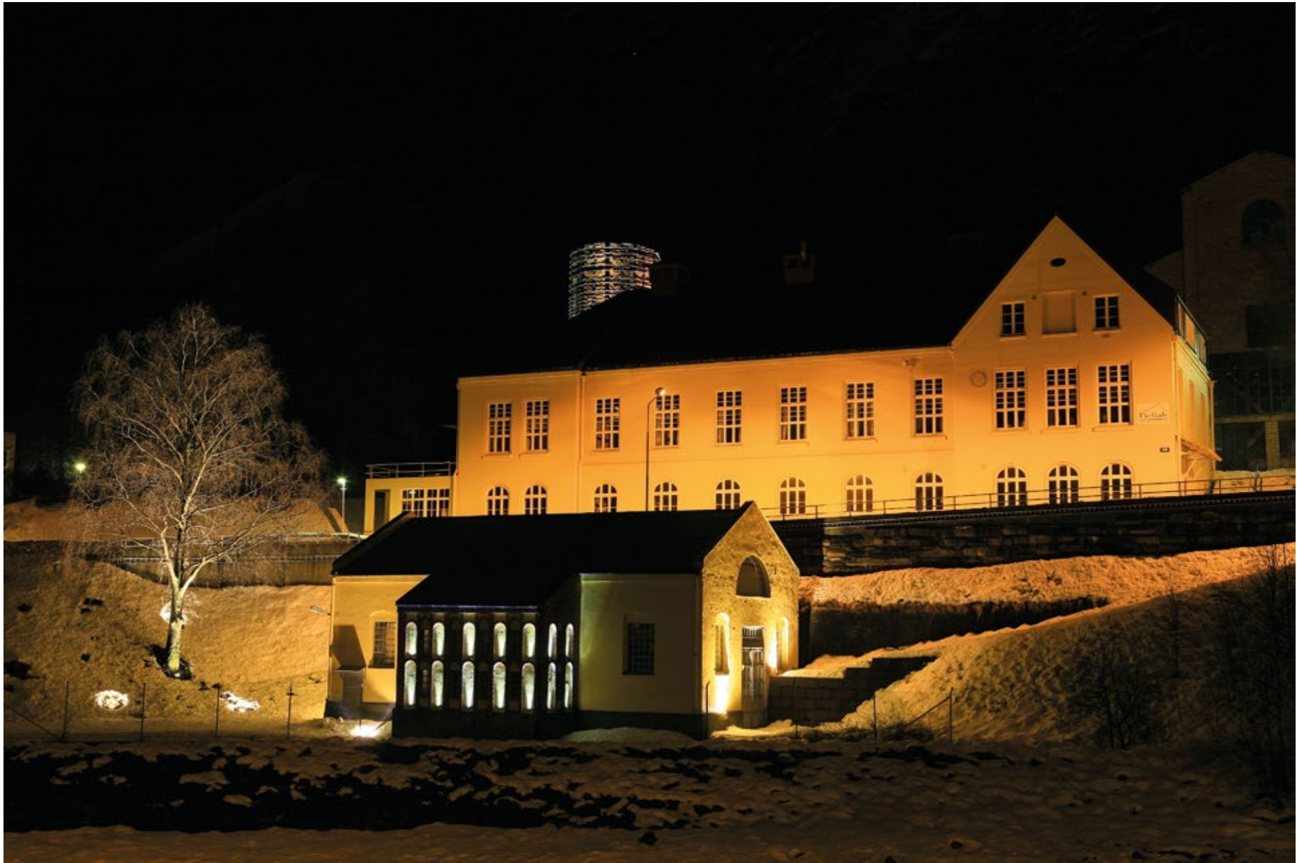
Fig. 61 Pump House, Laboratory and Acid Tower, Hydro Industrial Park in Rjukan Photo: Hans-Dieter Fleger
