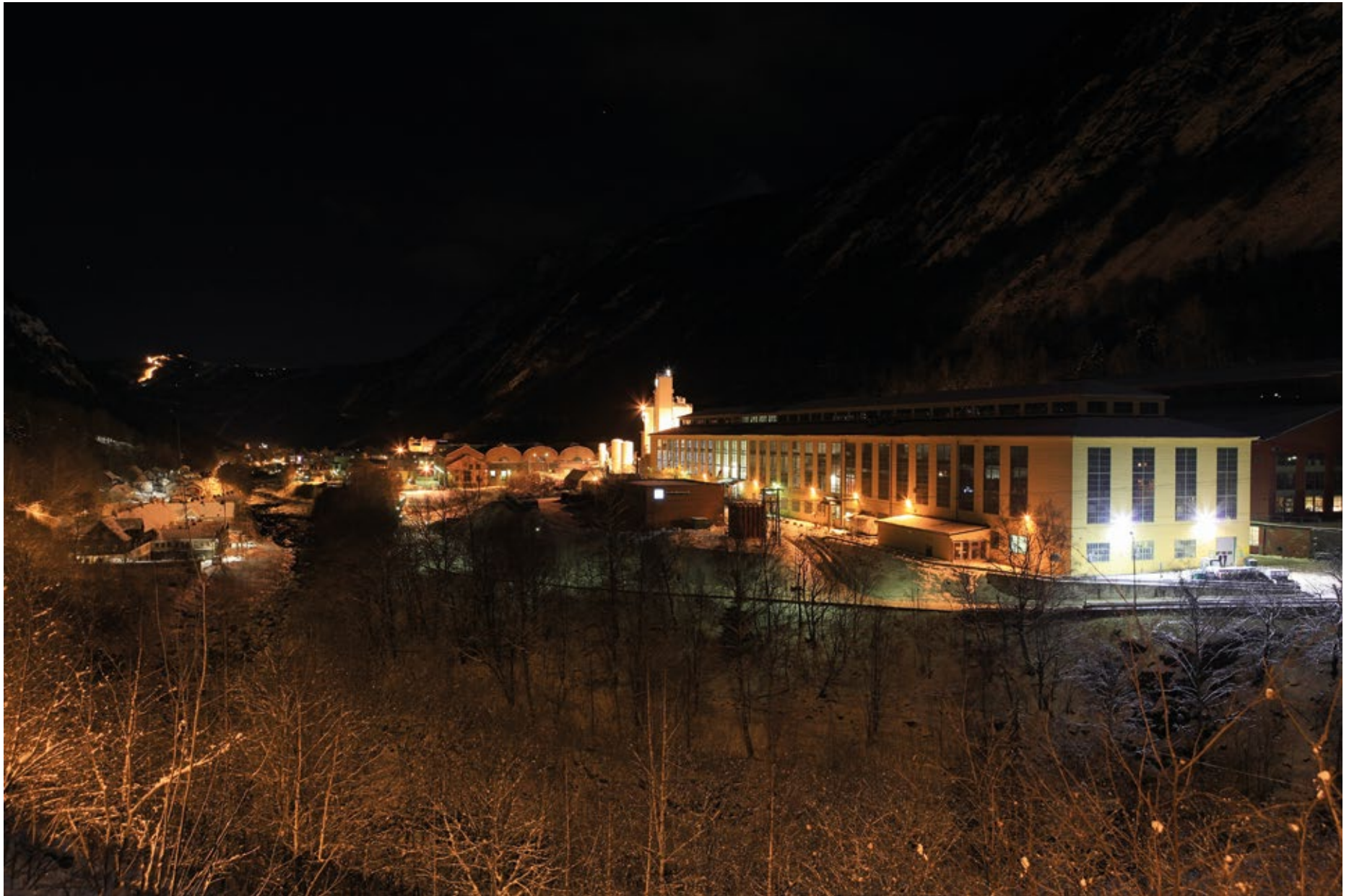
Fig. 56 Hydro Industrial Park in Rjukan facing east Photo: Hans-Dieter Fleger
