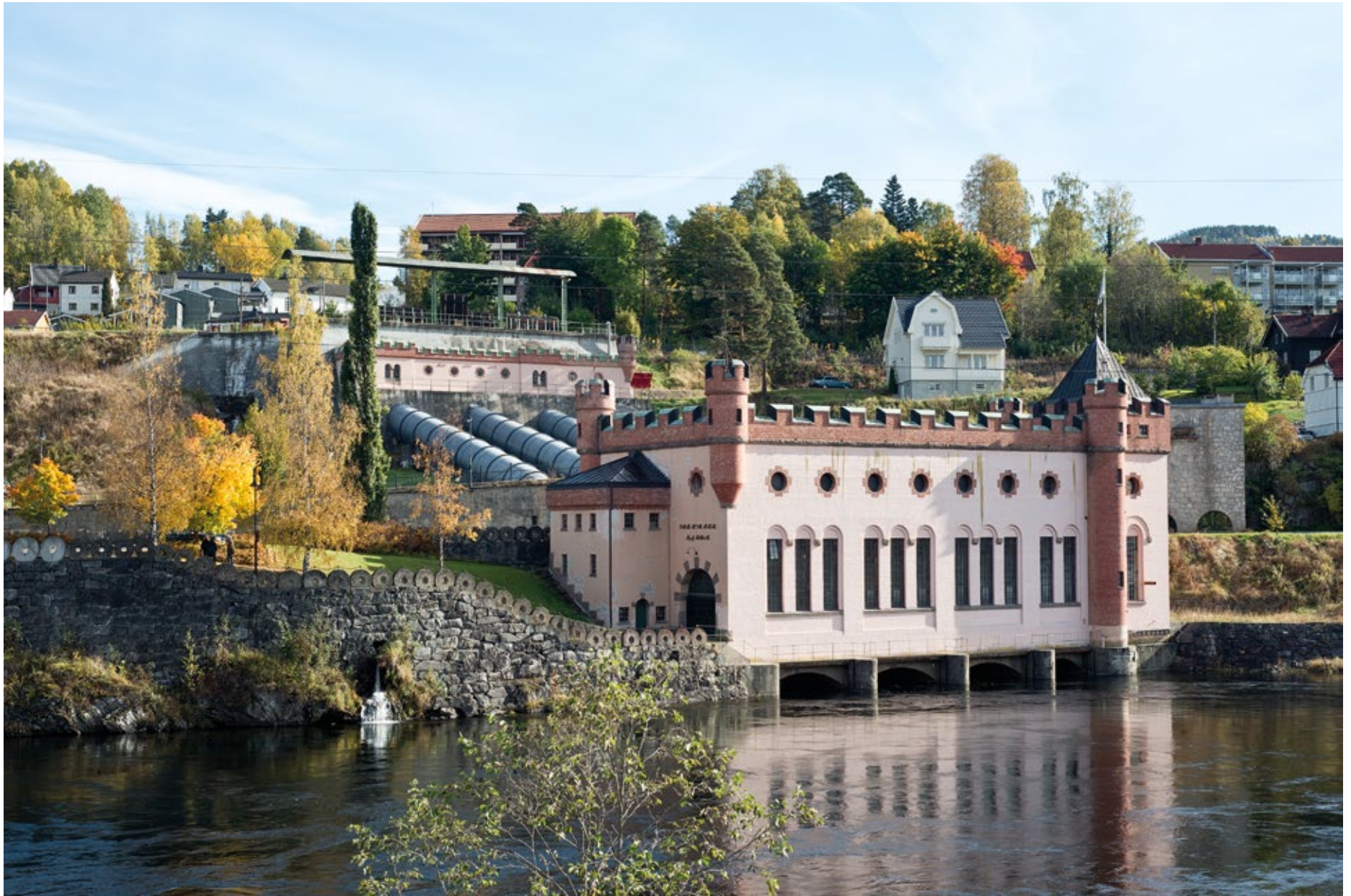
Fig. 12 Tinfos II Power Plant. Photo: Per Berntsen
