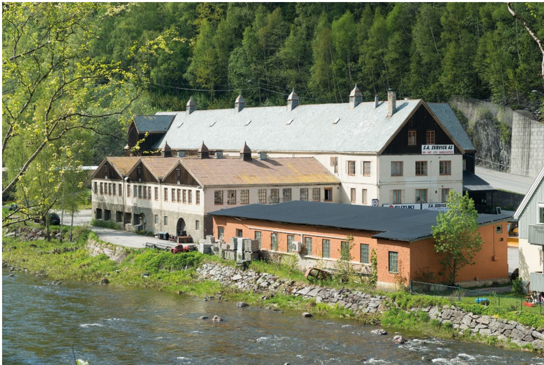
Fig. 96 Fjøset farm building, Rjukan Hydro Town. Photo: Per Berntsen
