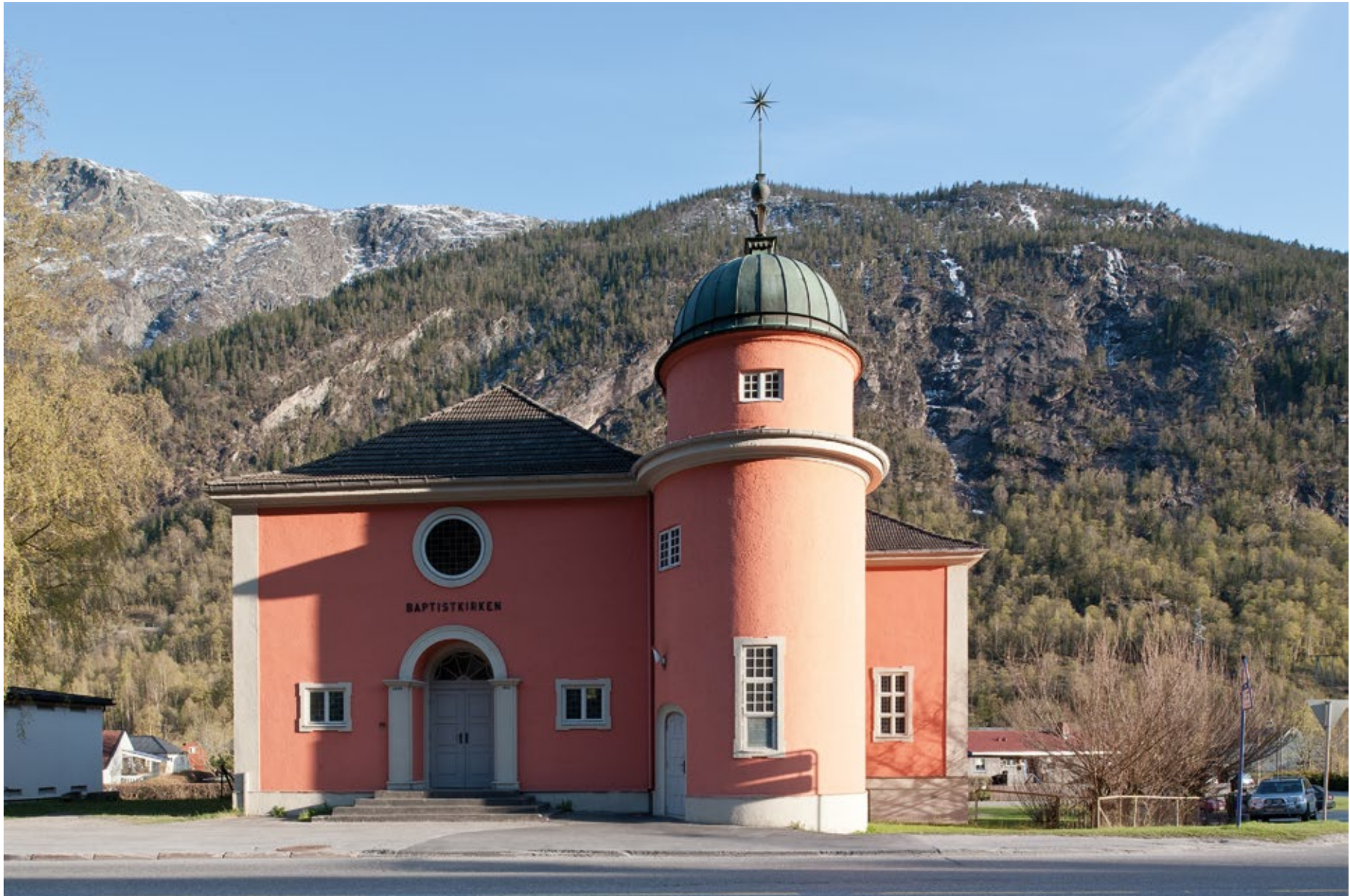
Fig. 107 Baptist Church, Rjukan Hydro Town. Photo: Per Berntsen
