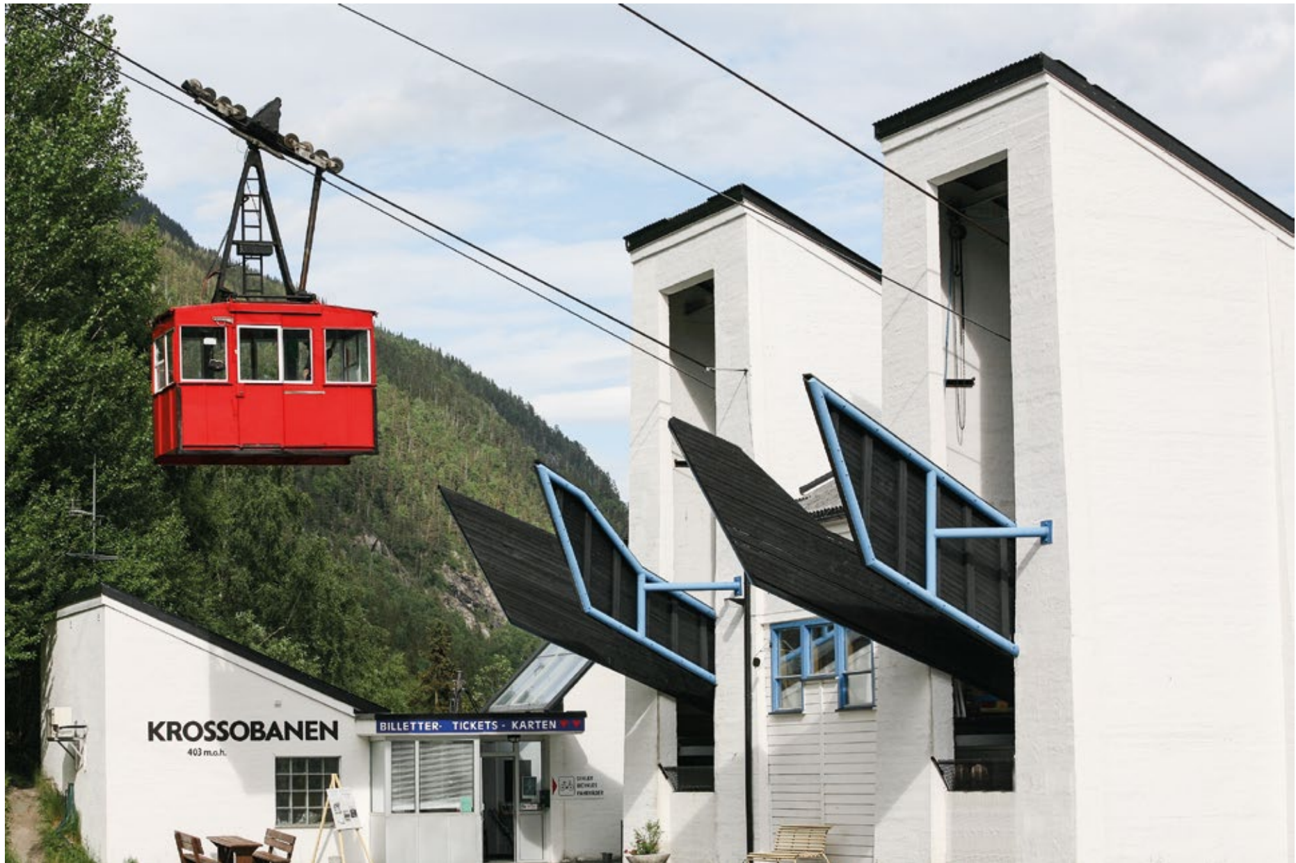
Fig. 93 Krosso Aerial Cableway, Rjukan Hydro Town. Photo: Hans Dieter Fleger
