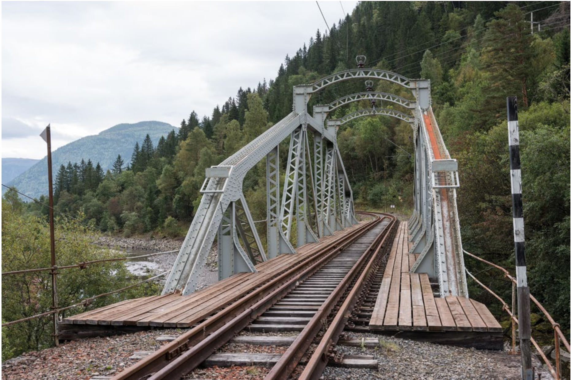
Fig. 81 Miland bridge, The Rjukan Line. Photo: Per Berntsen
