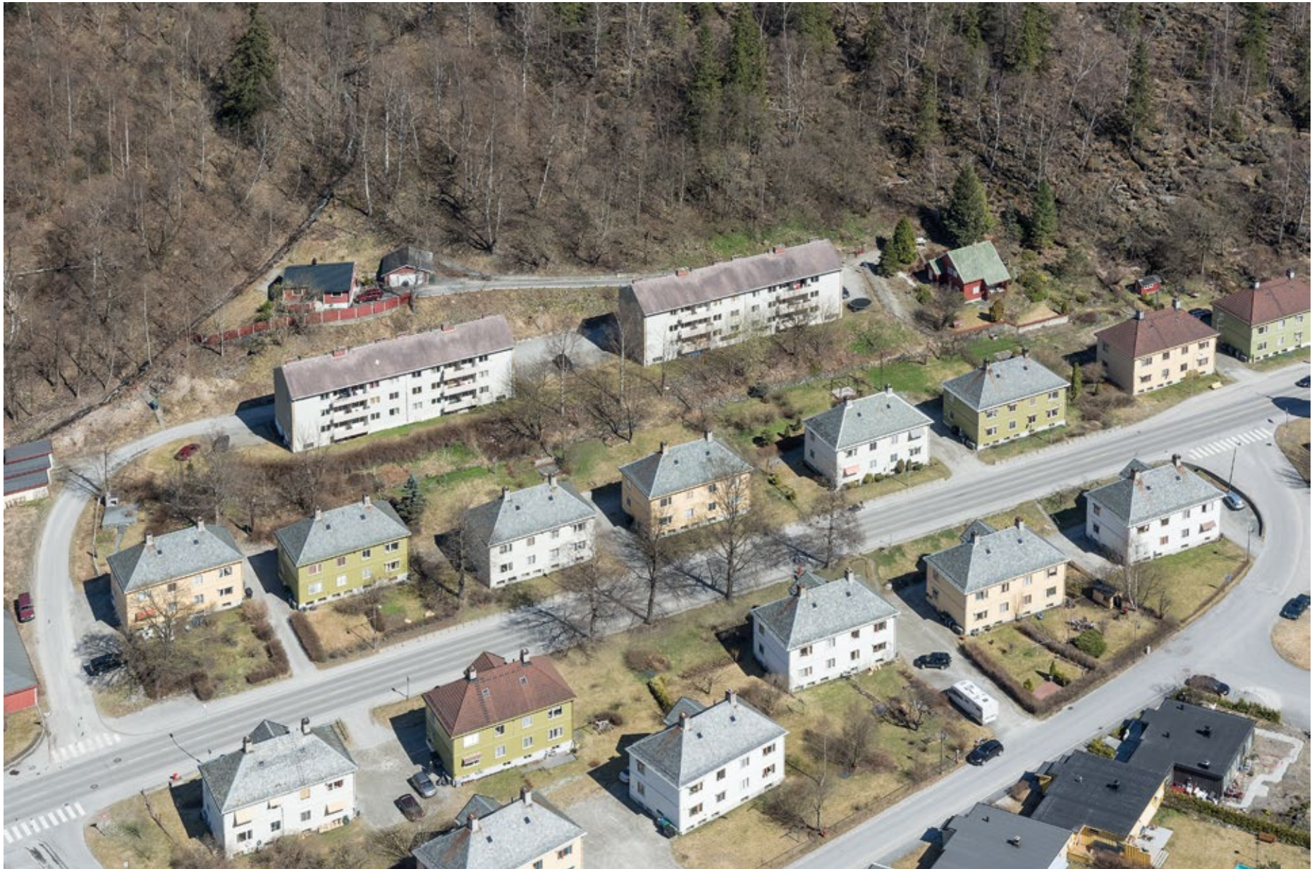
Fig. 105 New Town (house type O), Rjukan Hydro Town. Photo: Per Berntsen
