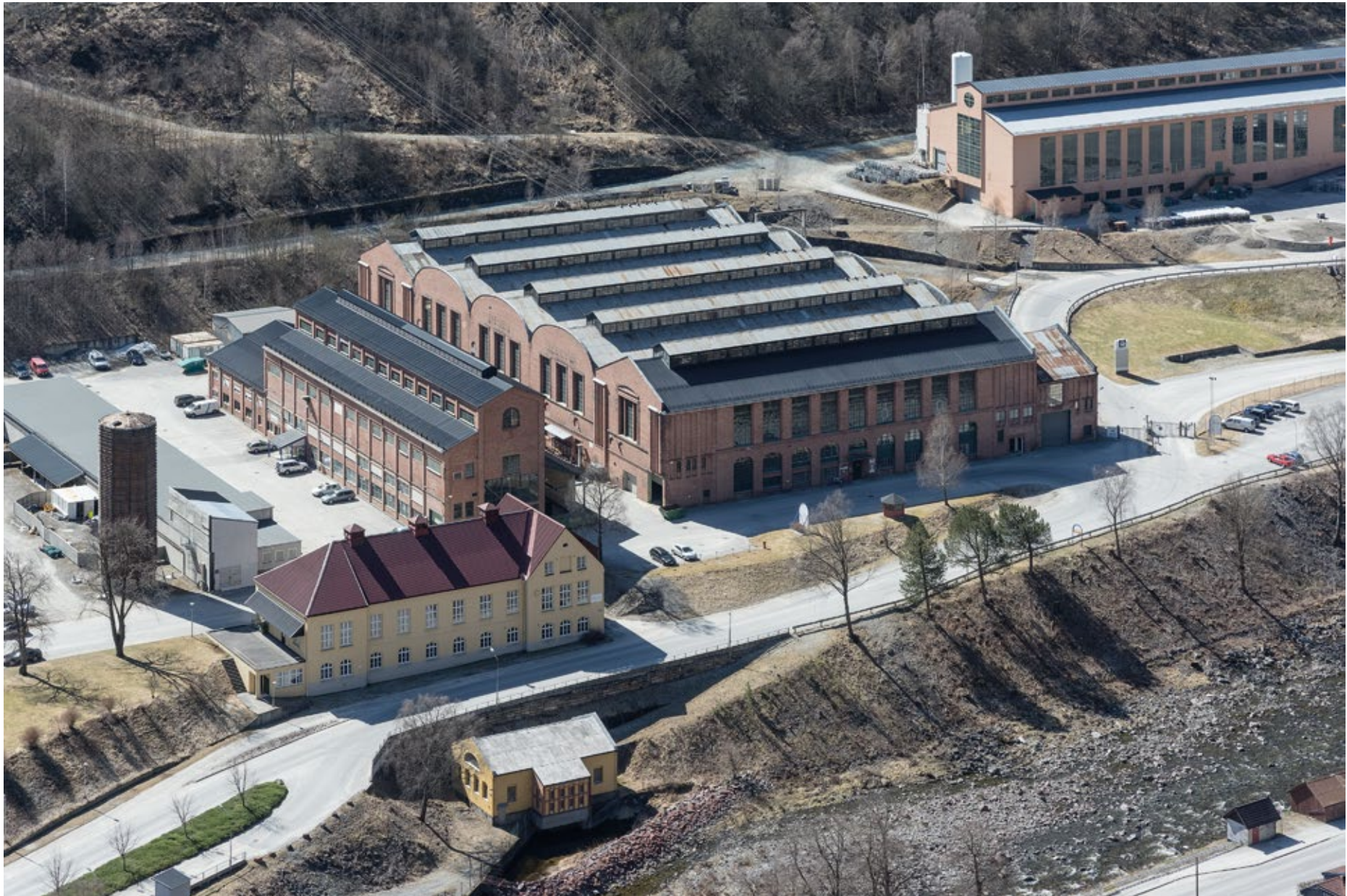
Fig. 57 Part of Hydro Industrial Park in Rjukan. Photo: Per Berntsen
