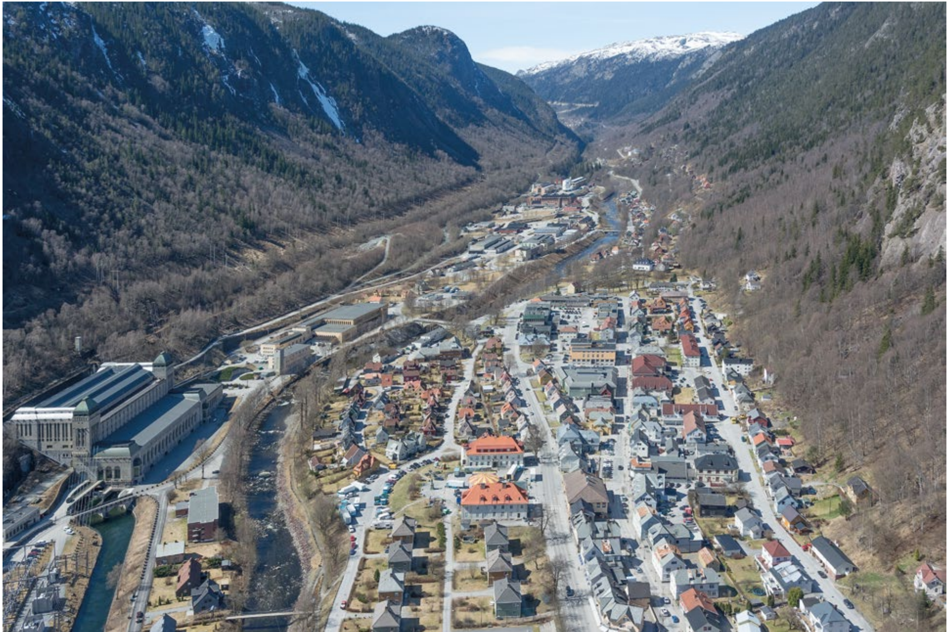
Fig. 110 New Town (house type O), Market Square and Tyskerbyen housing area facing west, Rjukan Hydro Town Photo: Per Berntsen
