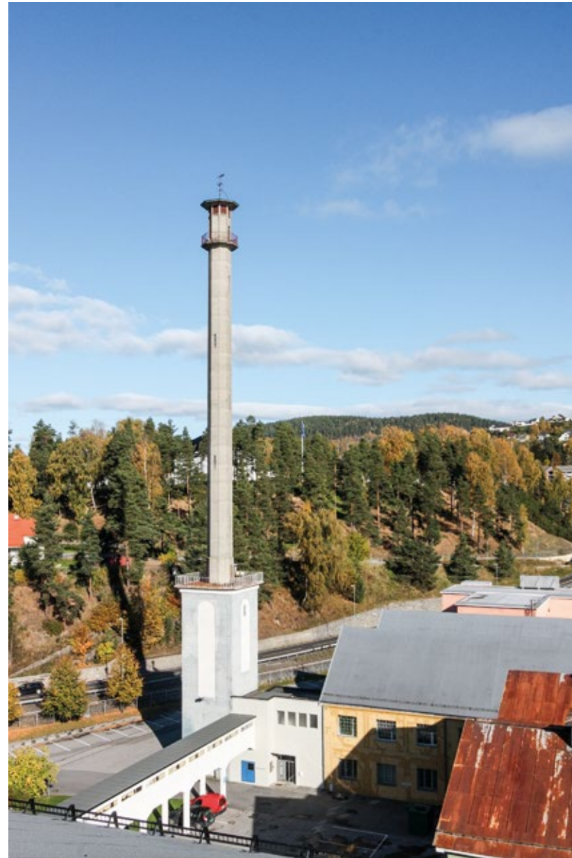
Fig. 49 The Minaret, Hydro Industrial Park in Notodden. Photo: Eystein M. Andersen
