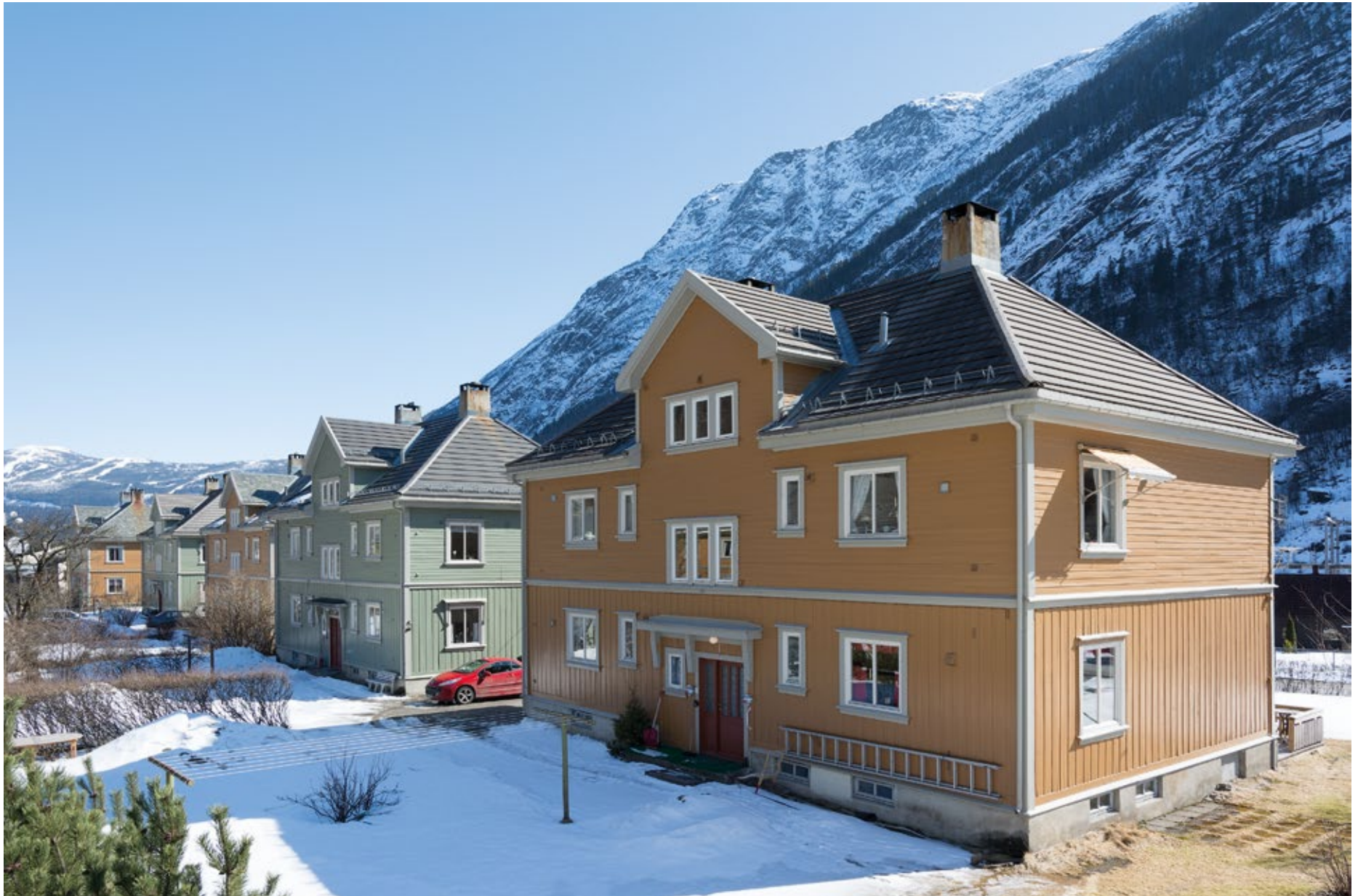
Fig. 106 New Town (house type O), Rjukan Hydro Town. Photo: Per Berntsen
