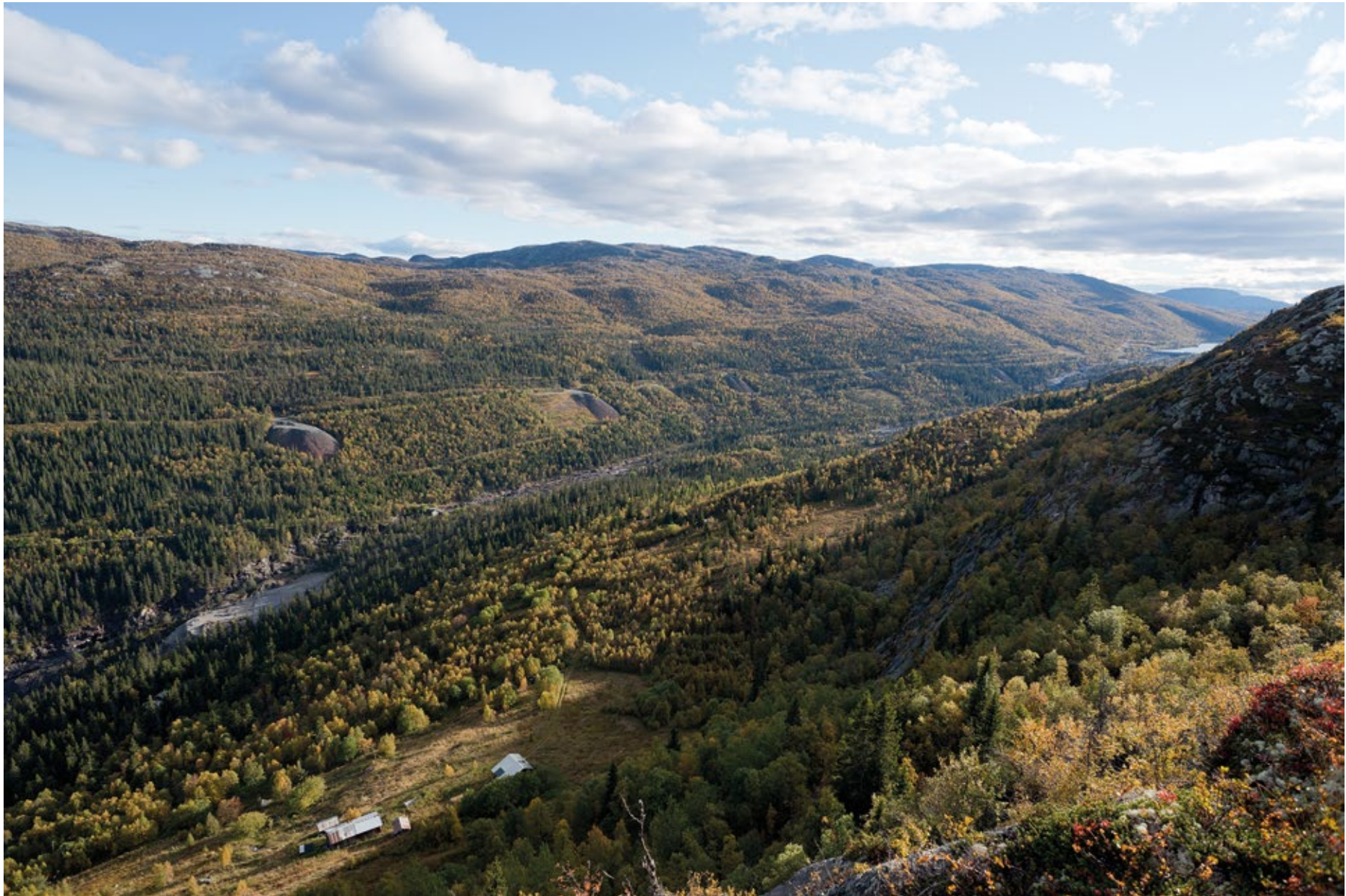
Fig. 19 Waste rock dumps between Skarsfos Dam and Vemork Power Plant. Photo: Per Berntsen
