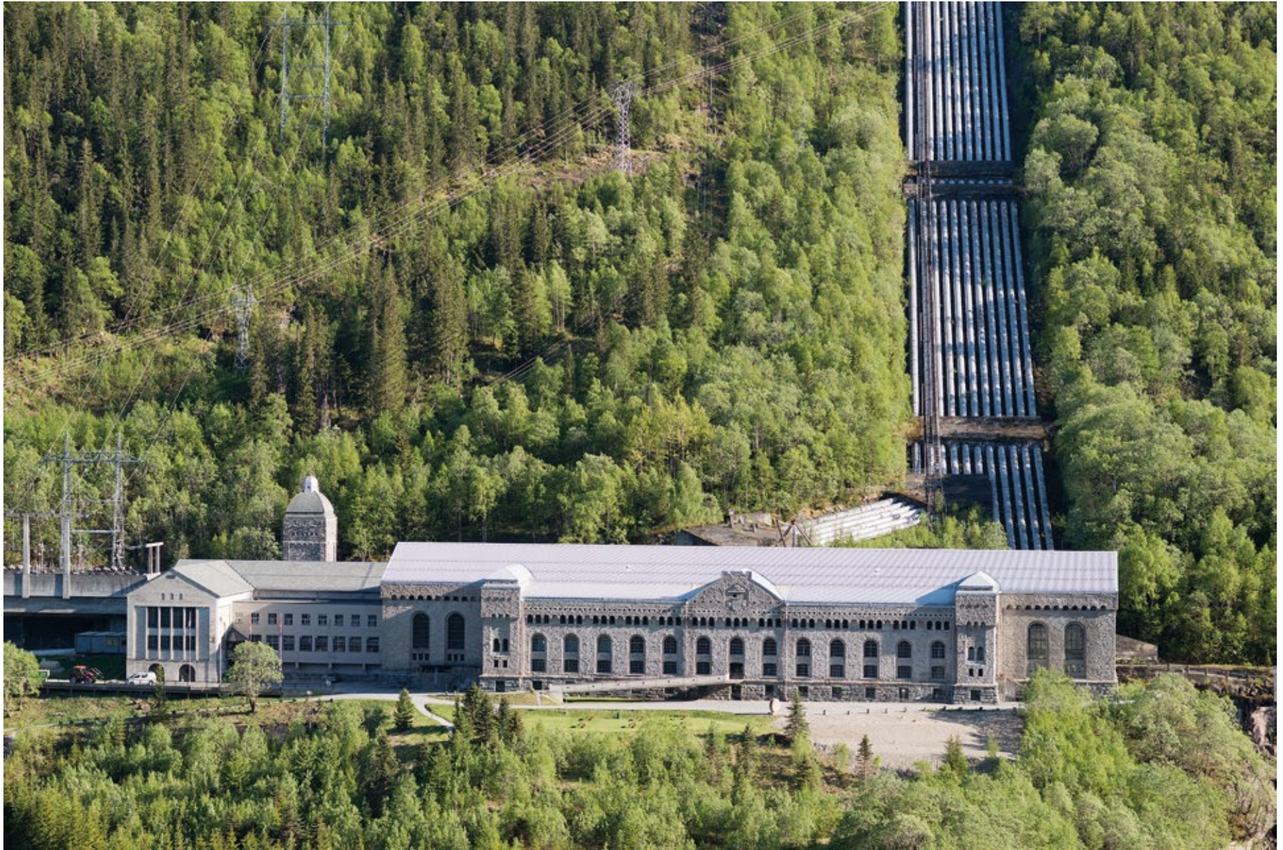
Fig. 24 Vemork Power Plant. Photo: Per Berntsen
