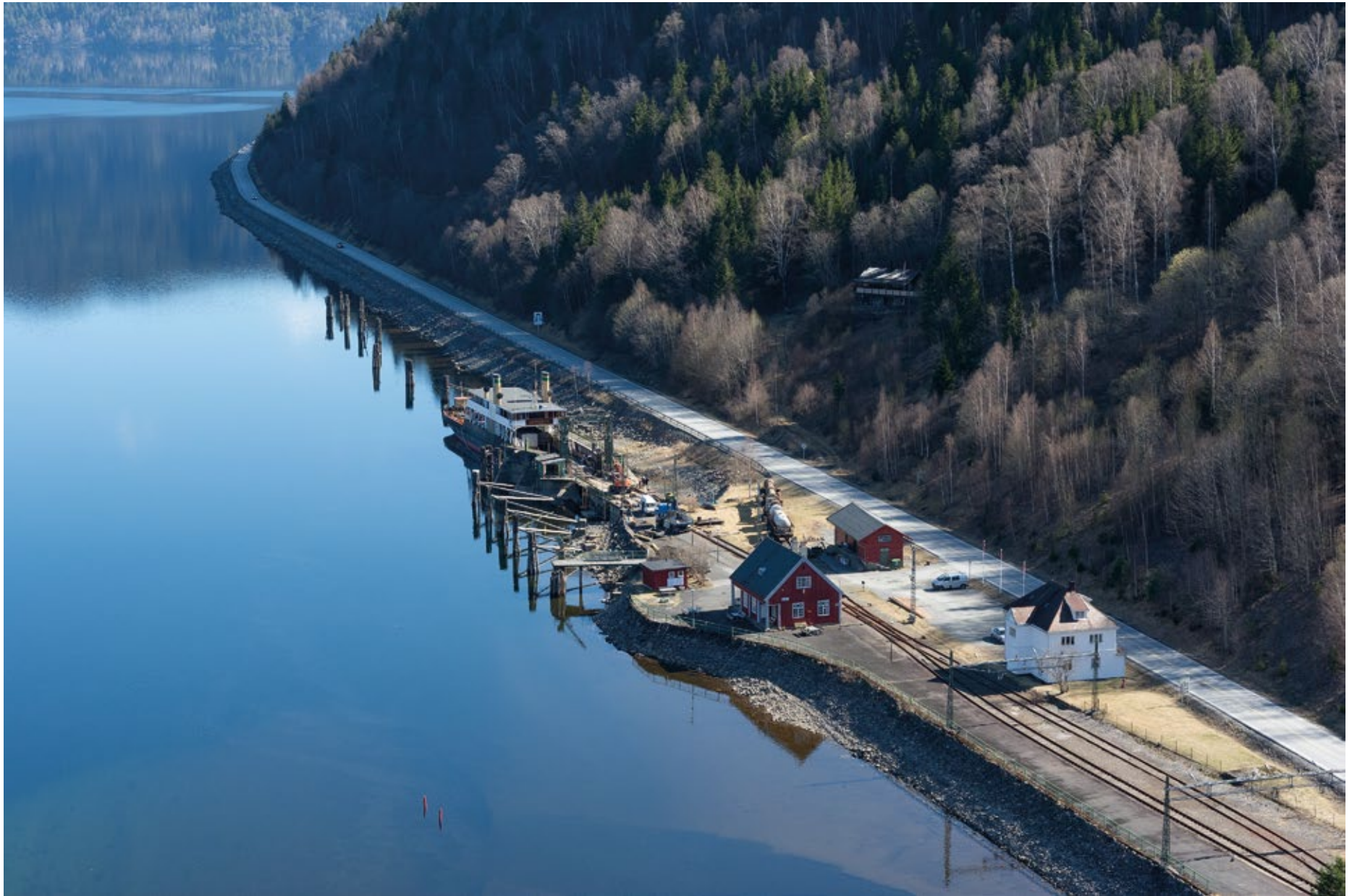
Fig. 78 Mæl Railway Station and Ferry Quay. Photo: Per Berntsen
