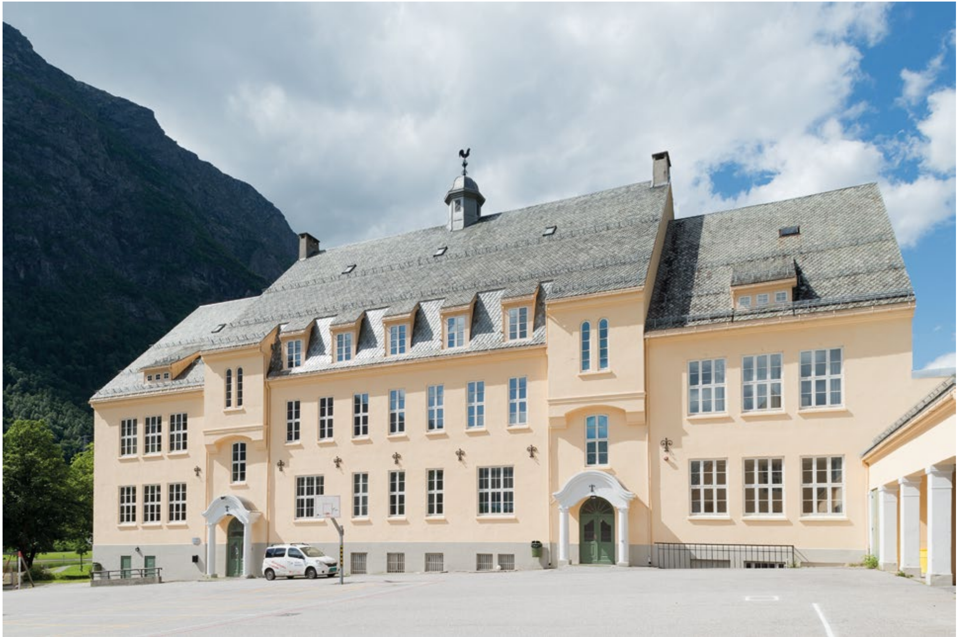
Fig. 115 Tveito School, Rjukan Hydro Town. Photo: Per Berntsen
