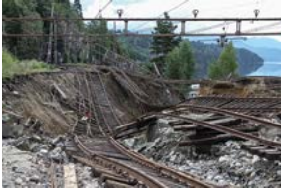
In summer 2011, large parts of Notodden railway station was washed away, when the stream found a new course during a flood after prolonged period of rain. The area was rebuild and flood protection improved. Left photo: Unn Yilmaz. Right photo: Eystein M. Andersen.
