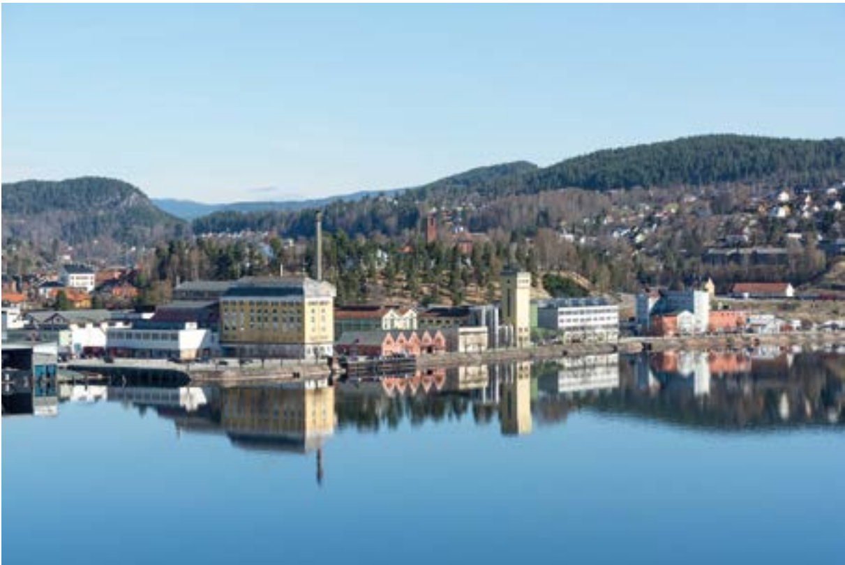
Hydro Industrial Park in Notodden facing north east. Photo: Per Berntsen.
