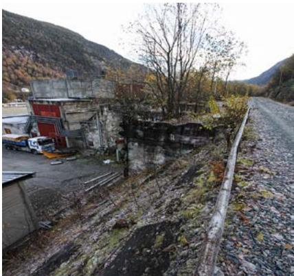
Remains of the dissolution plant in Tower House I. Photo: Eystein M. Andersen.
