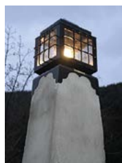
Original lighting on Birkeland Bridge, restored in 2012. Photo: Bjørn Iversen.
