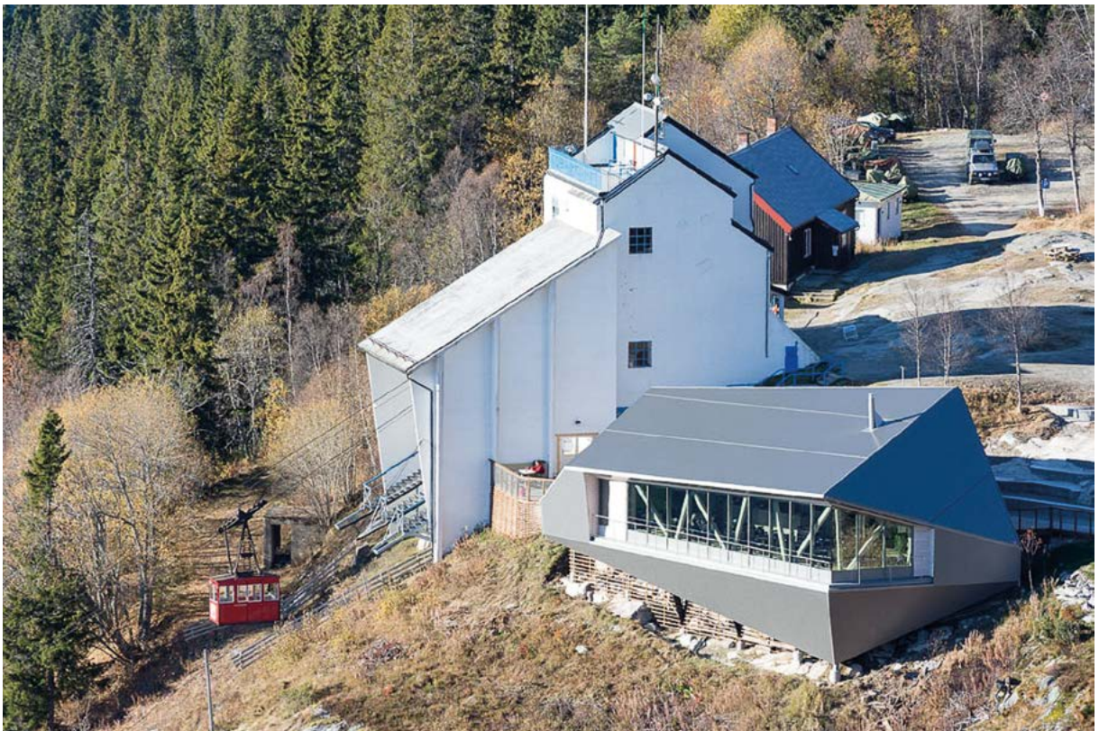
The new café at Gvepseborg on the top station of Krosso Aerial Cableway. Photo: Per Berntsen.
