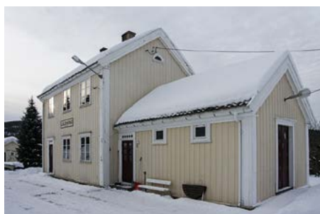
Lisleherad station building. Photo: Eystein M. Andersen.
