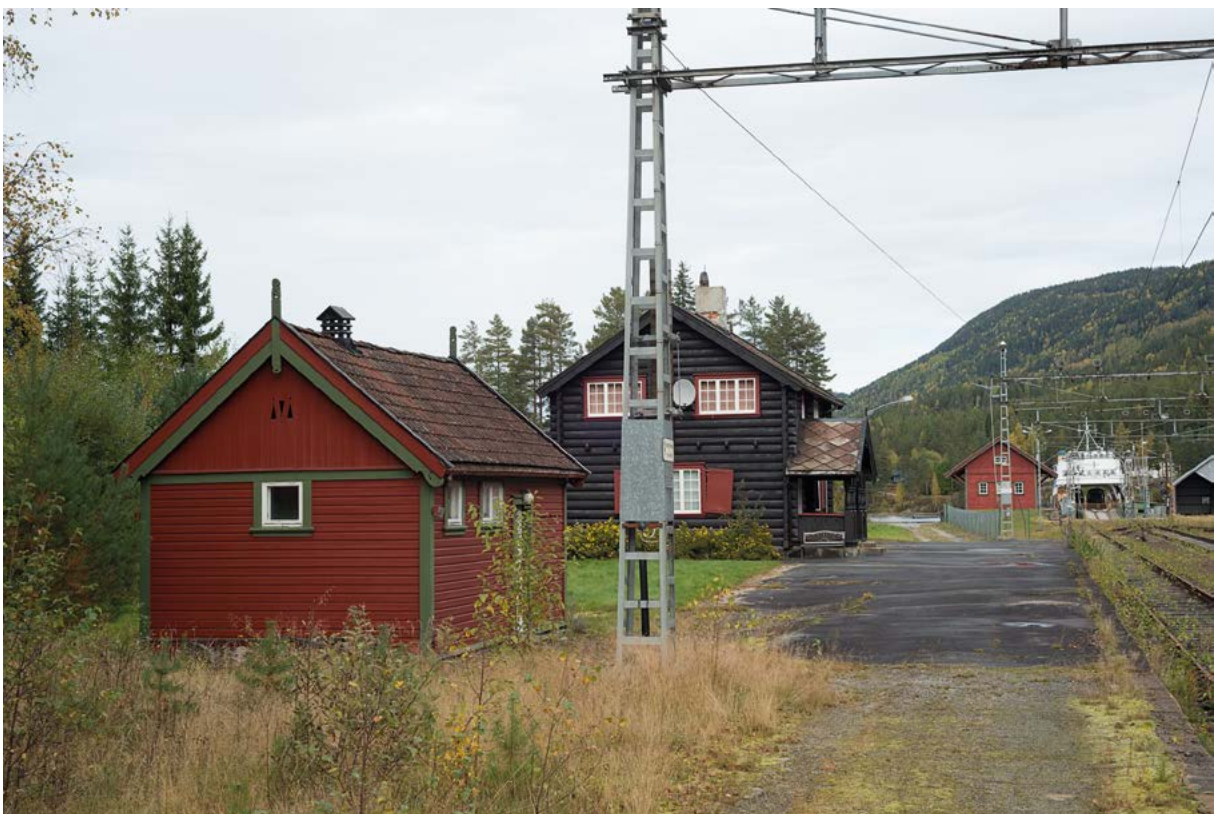
Tinnoset Railway Station with three buildings, the outhouse in front. Photo: Per Berntsen
