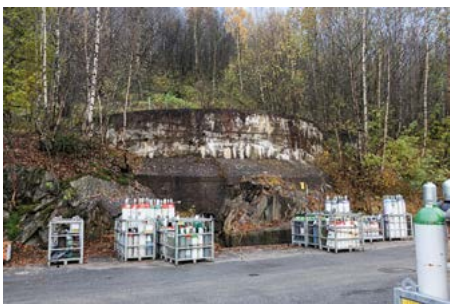
Remains of the gasometer for ammonia. Photo: Eystein M. Andersen.
