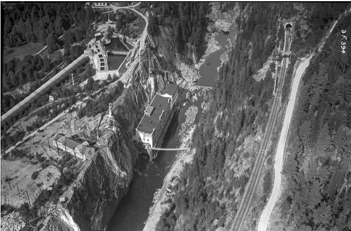
Svælgfos mid 20th century with the power station in the gorge and the lightning arrester house on the cliff. The Tinnoset line to the right.
