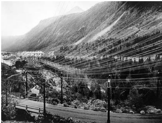
Power transmission from Vemork to the industry area in 1912. Photo: Anders B. Wilse.
