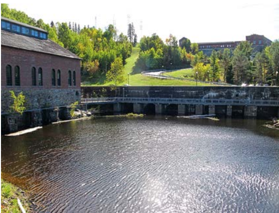
Shawinigan in Quebec, where the generator floor and water outlets remain from the Shawinigan I power plant, besides the power house building of Northern Aluminum Co (left) that is now part of a theme park on electricity. Photo: Trond Taugbøl.
