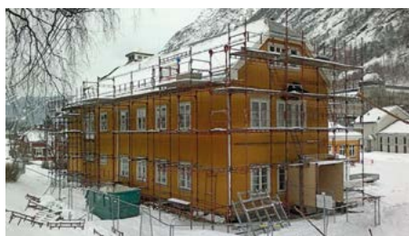
Såheim private school under restoration in 2013. Photo: Bjørn Iversen.
