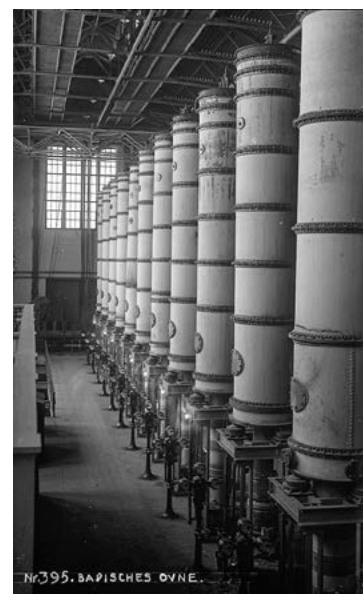
Furnace House I in 1910 to the left and part of its interior with Schönherr furnaces a few years later to the right. Photos: Norwegian Industrial Workers Museum.
