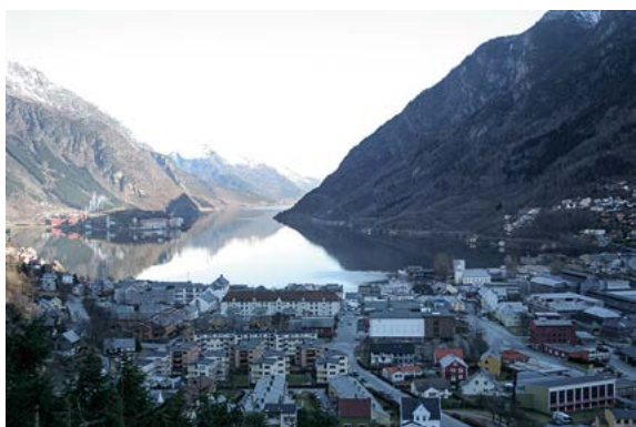
Odda industrial town with the Smelteverk to the right. There has been three, and still are two, industrial complexes located around the inner end of Sør fjorden, all harnessing the nearby waterfalls. Photo: Turid Årsheim, Riksantikvaren.
