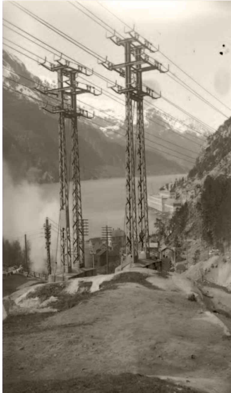
High-voltage power masts at Tveit near Tyssedal, 1915. The factories in Odda and Tyssedal got their electric power from the Ringedal water system, which drained a number of large and small lakes in the south-western area of the Hardanger Plateau. From the shoreline power station, AIS Tyssefaldene (in the background), the 12,000 volt current was transported over 6-7 kilometre-long cables, which were laid out in 1906-08 and 1909. They were in use until 1995. Photo: AIS Tyssefaldene. Norwegian Museum of Hydro Power and Industry.
