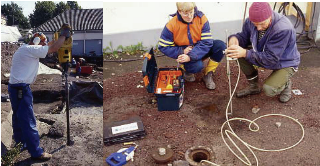
Left: installation of a dipwell, using a manual drilling rig; right: taking a water sample from a dipwell (photos: NIKU).
