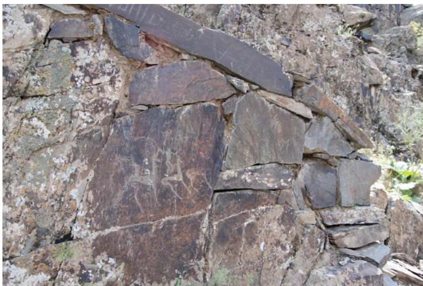
Protective works on Group IX (cf. photo in the Norwegian report from 2007, page 15). Photo: A-S Hygen
