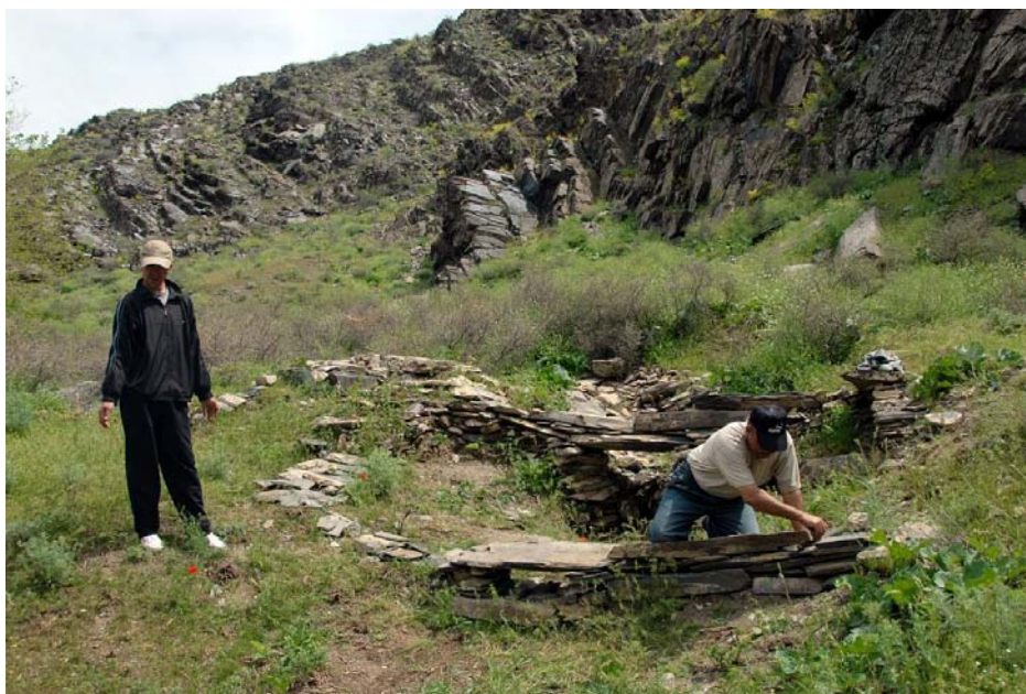
Work is underway to restore an old water mill (route 2, point 7).
