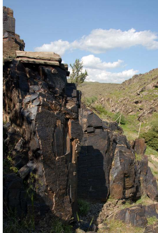
The small slab roof over group VII.
