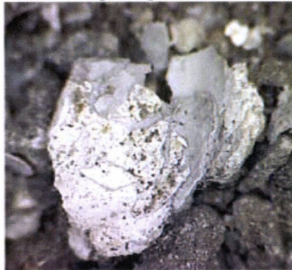
Plate 5. Close up of a loose shell-lime inclusion within the mortar fines (c. x50 magnification).
