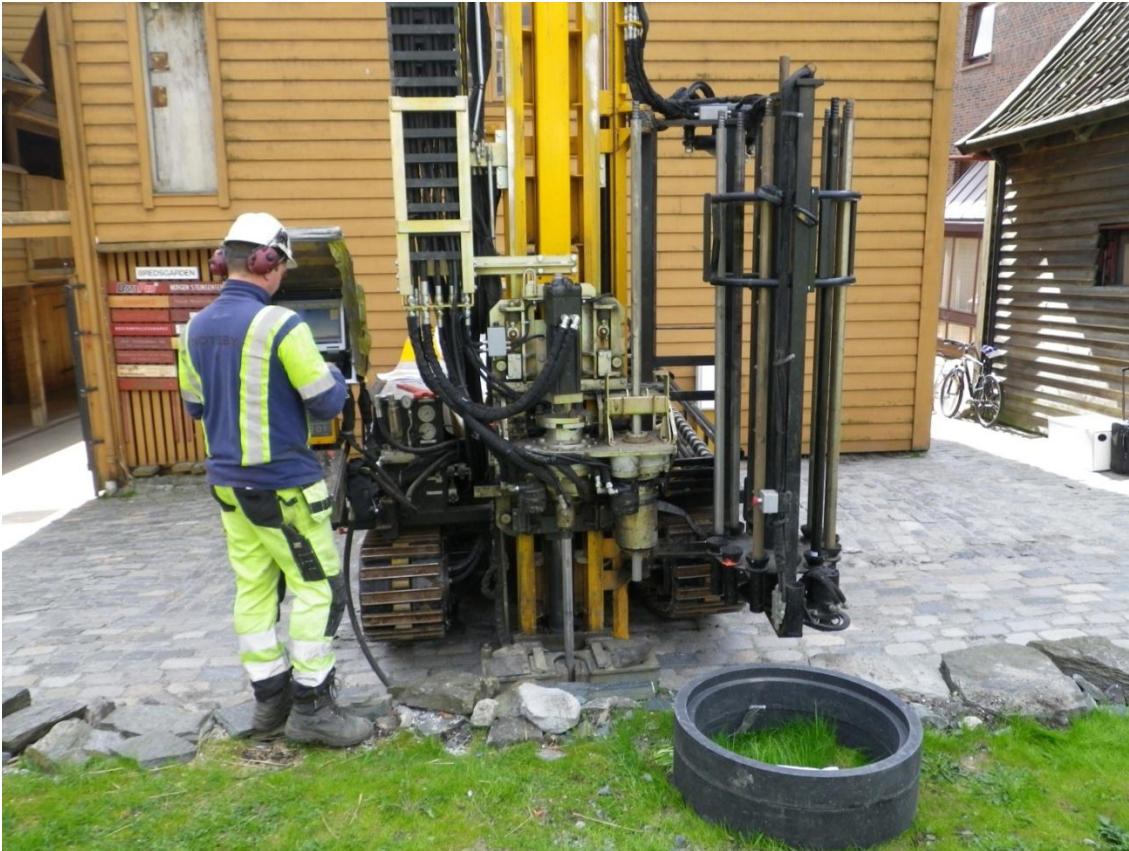
Figure 3: Picture of the rig with gauging probe (Direct Push technique)
