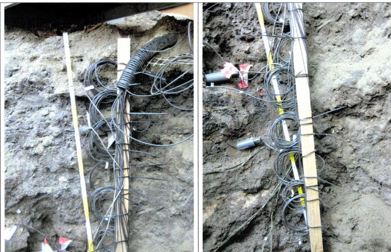
Figure 3: South-east profile of testpit after installation of sensors. The picture to the left shows the upper strata (ca 3.1-4.1 m asl), whereas the picture to the right shows the lower strata (ca 2.25-3.3 m asl) – the deepest lying sensors at 2 m asl are not visible.
