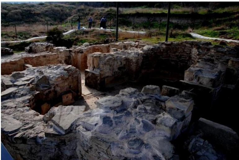
*Masonry work at one of the ruins at Bagineti Acropolis. Only lime mortar is now applied.*
