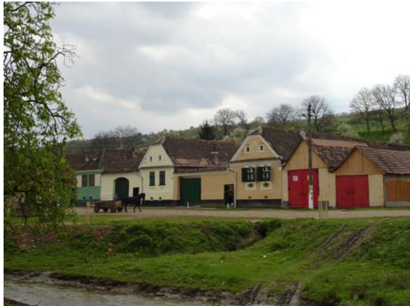
Restored house fronts Malencrav - Malmkrog. © Riksantikvaren
