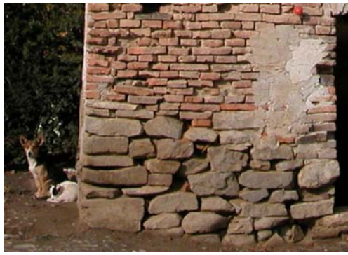
A quite normal pre work condition. Detail of cold wall at the base of the house with overlaying brick wall. © Riksantikvaren
