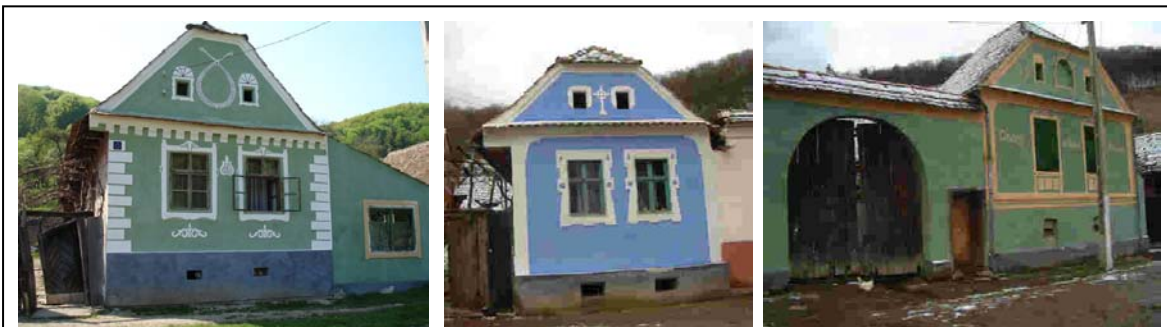
Houses Floresti – Felsenthal. © Riksantikvaren
